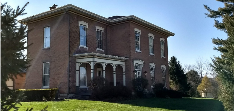
1. Main house at 5281 Brand Road from the northeast.
