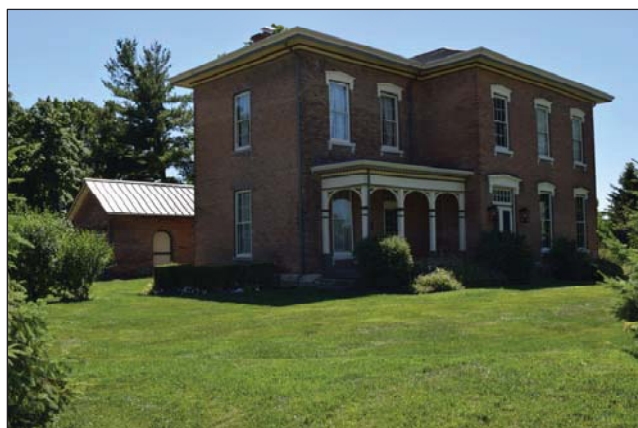
5281 Brand Rd, looking southwest
