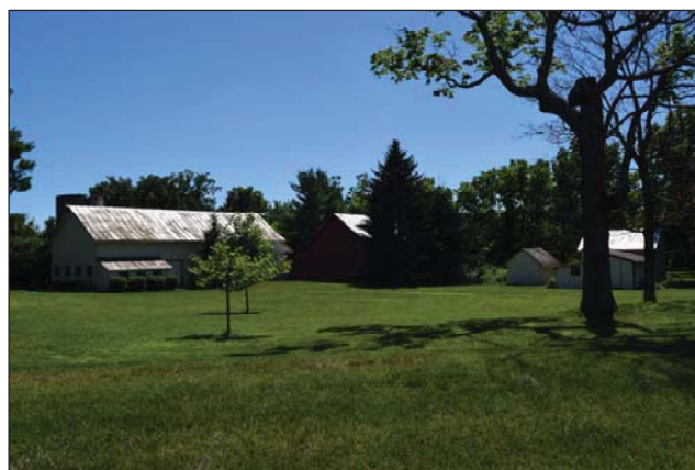
5281 Brand Rd, looking southwest
