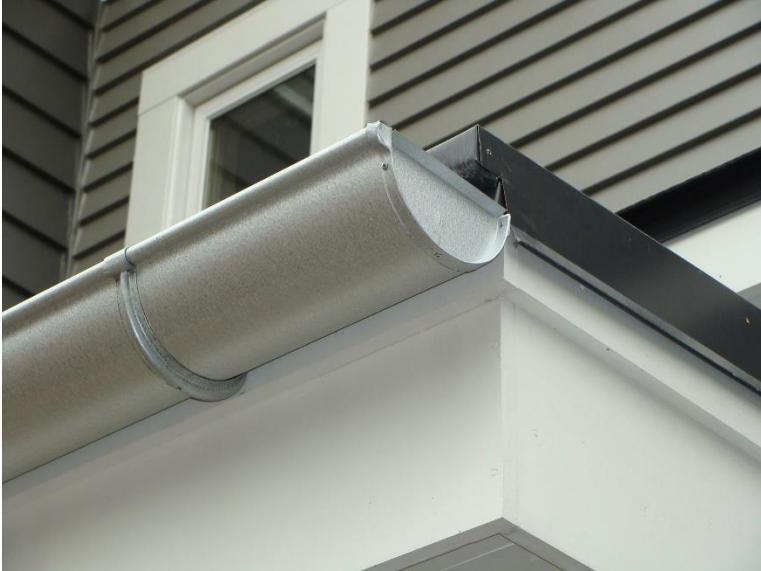
Gutter-half round Galvalume, round downspouts.
