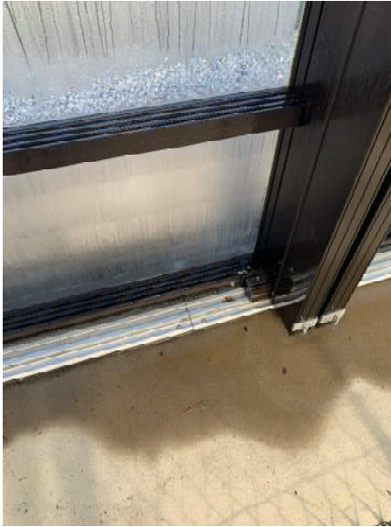
Interior Rail Detail
