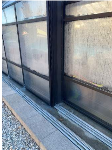
Interior Rail Detail
