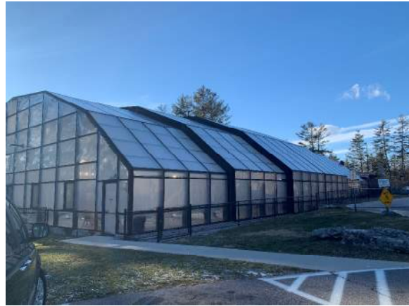
Exterior Day View
