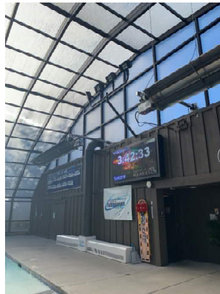
Interior Mechanical and Lighting
