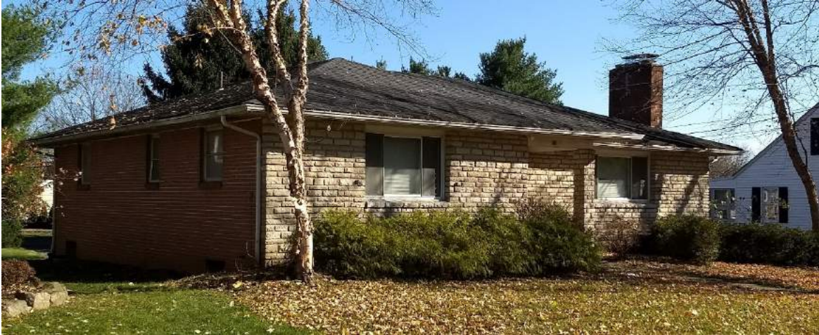
1. Ranch-style house at 86 Franklin Street from the northwest.
