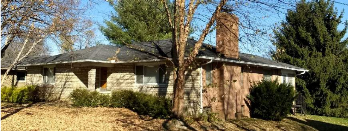
2. House at 86 Franklin Street from the southwest.
