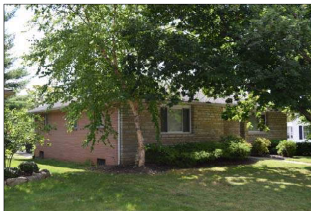
86 Franklin St, looking southeast
