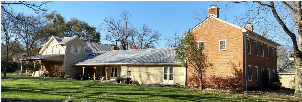
2. Photograph of 109 S. Riverview Street from the southeast.
