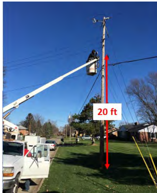
Figure 17. Bucket truck used to measure the Rx signal level at the approximate AP location.
