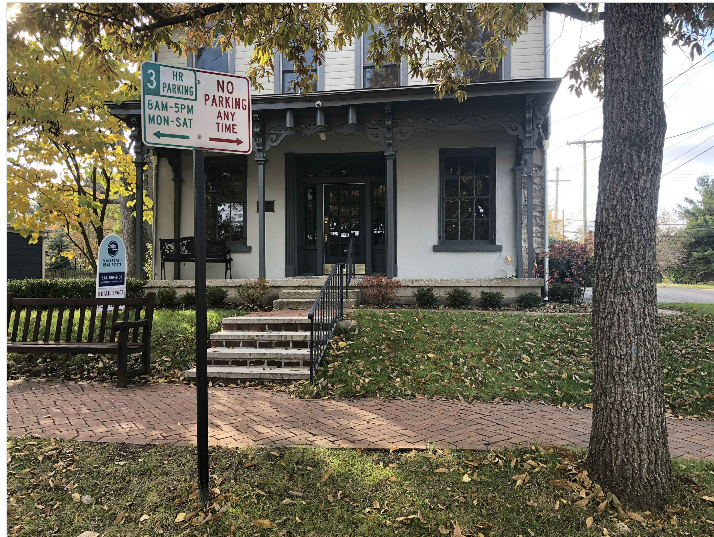
VIEW FROM DUBLIN ROAD (EAST SIDE)
