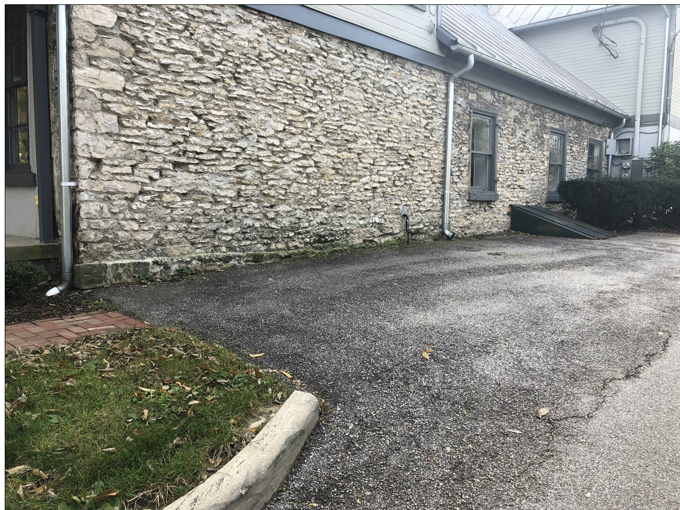
VIEW FROM EBERLY LANE (NORTH SIDE)
