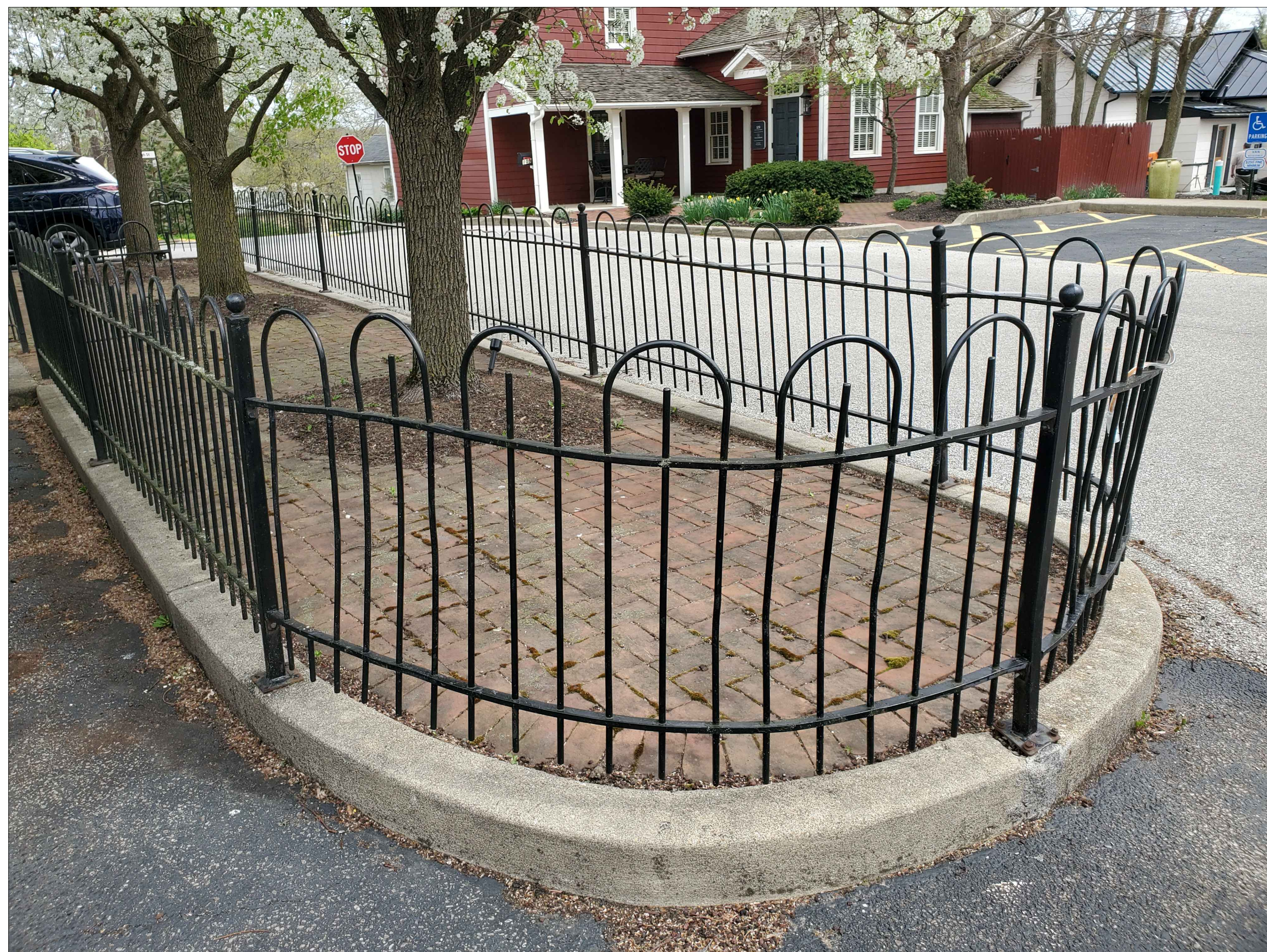
WROUGHT IRON RAILING EXAMPLE
