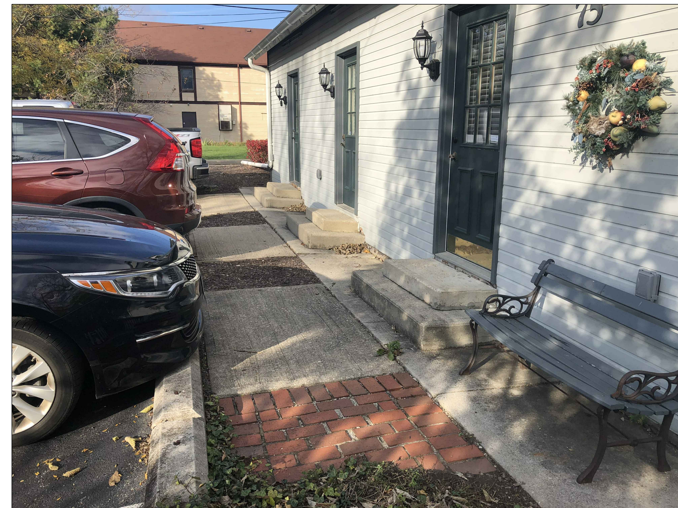
VIEW OF WEST SIDE (PARKING LOT)
