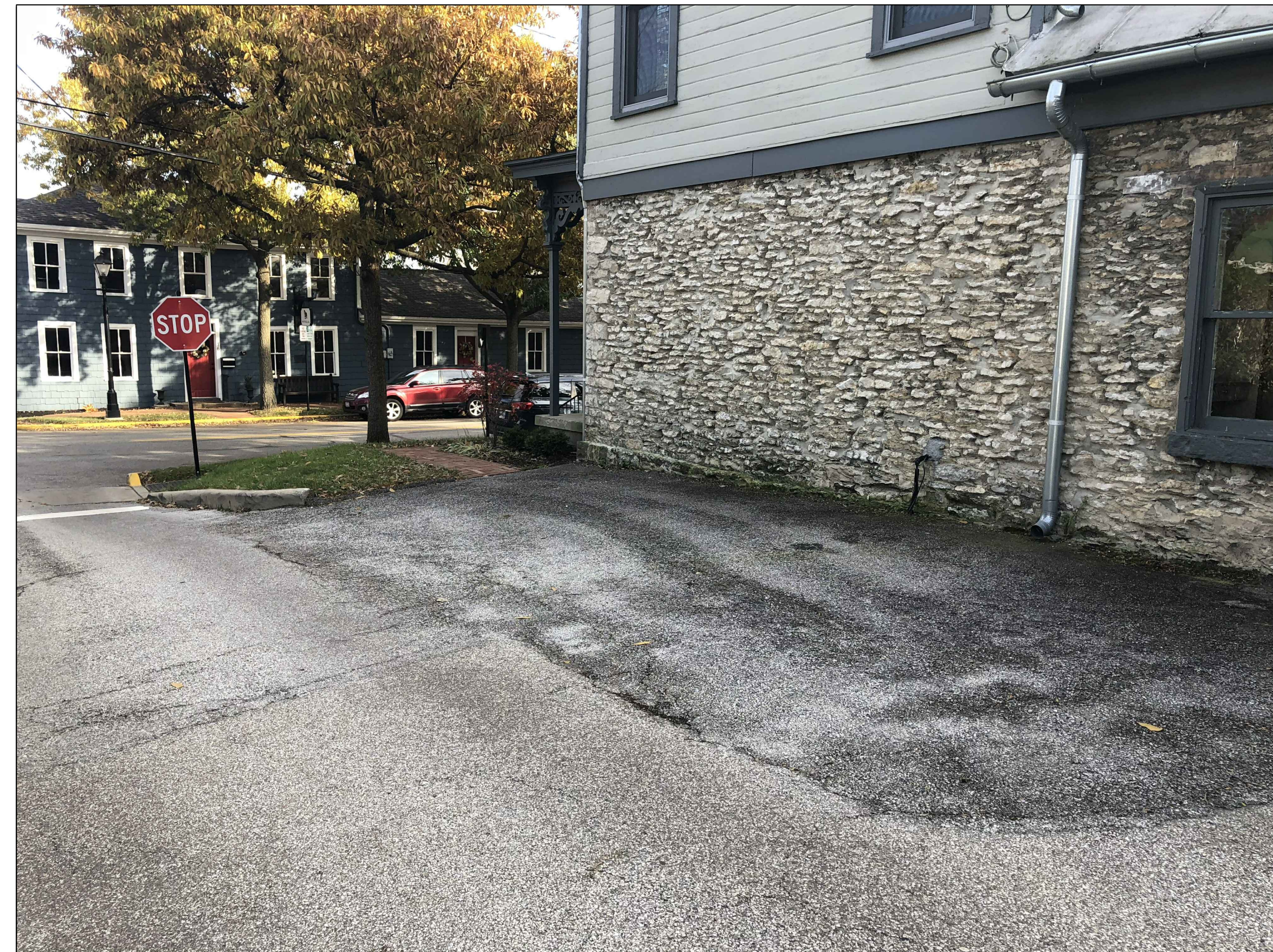
VIEW FROM EBERLY LANE (NORTH SIDE)
