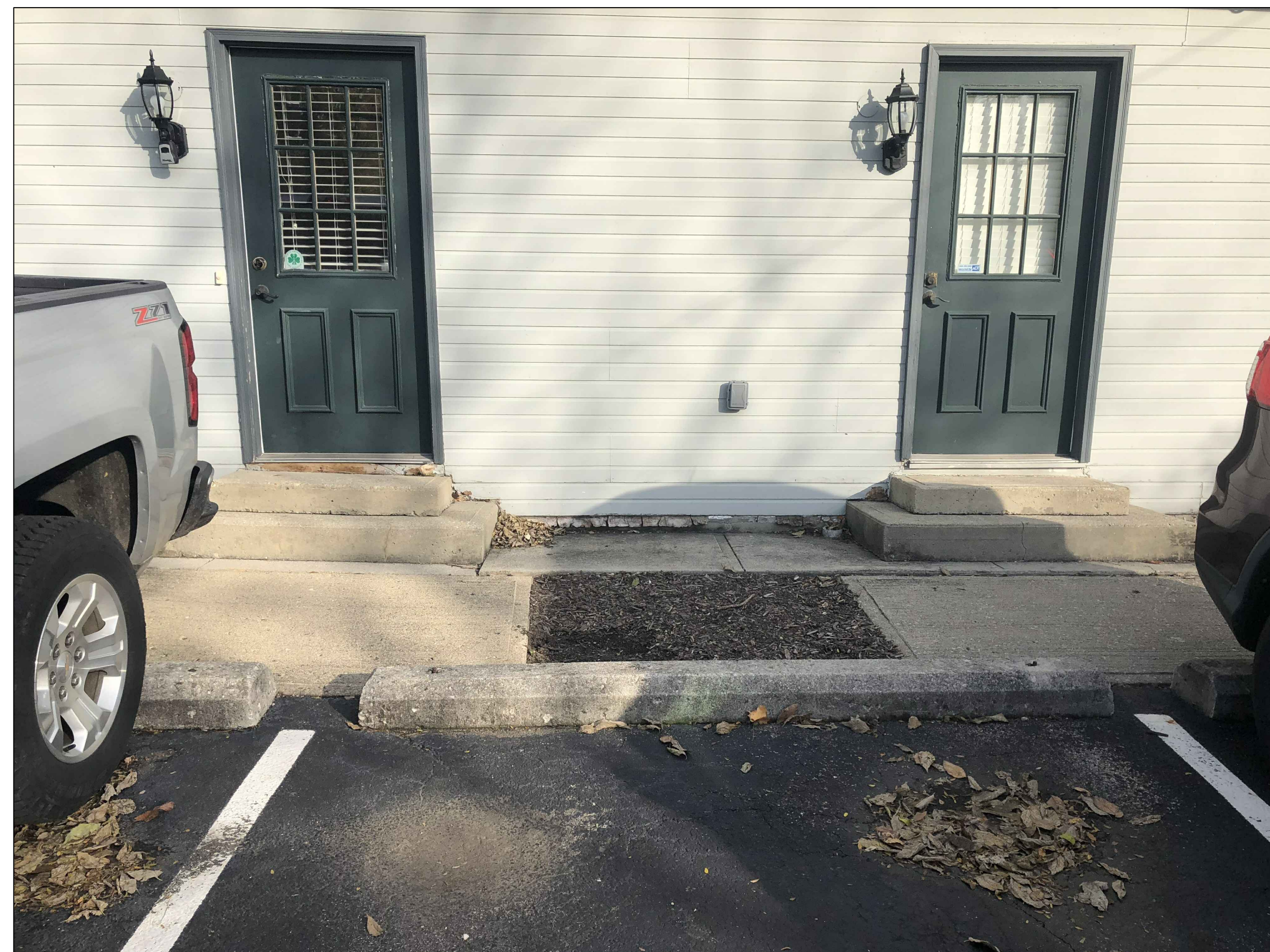
BACK STEP DETAIL IMAGE (WEST SIDE)
