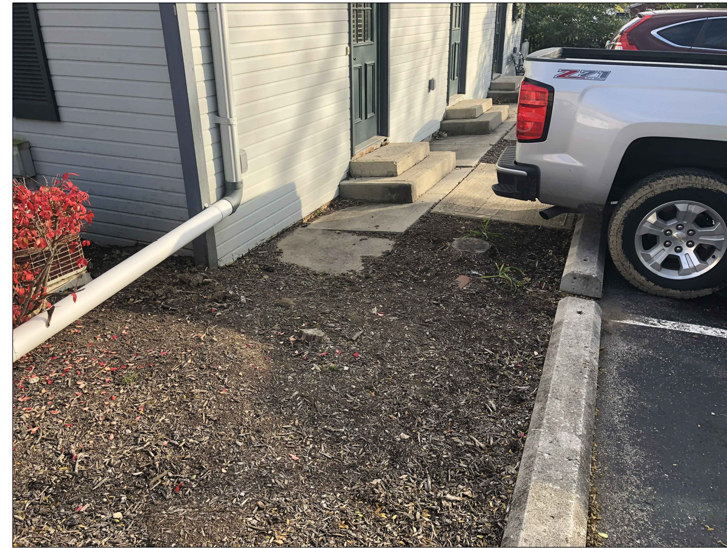
BACK STEP DETAIL IMAGE (NW CORNER)
