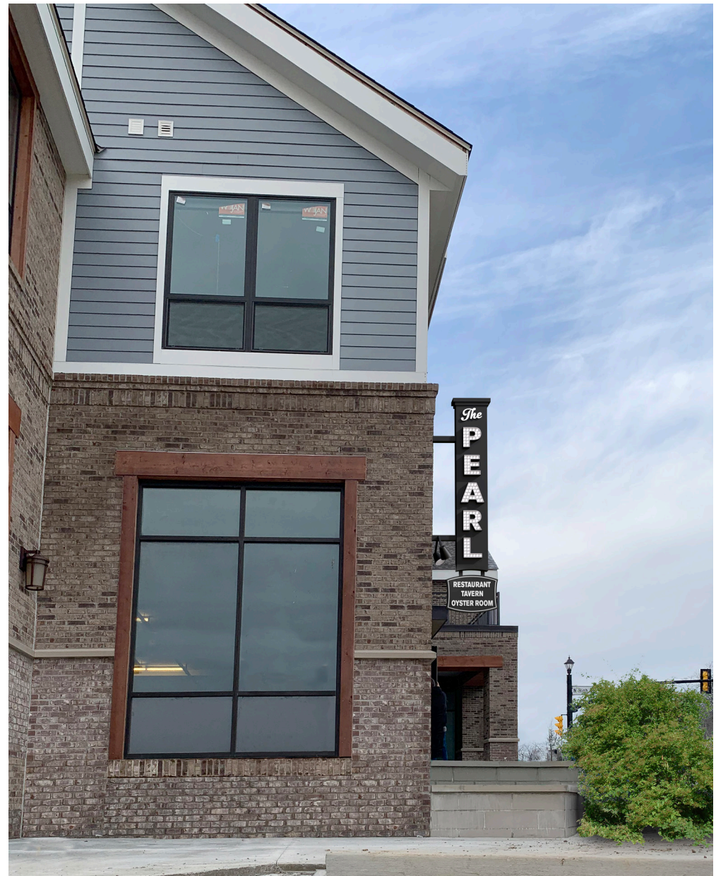
West Facing | Day Time View
