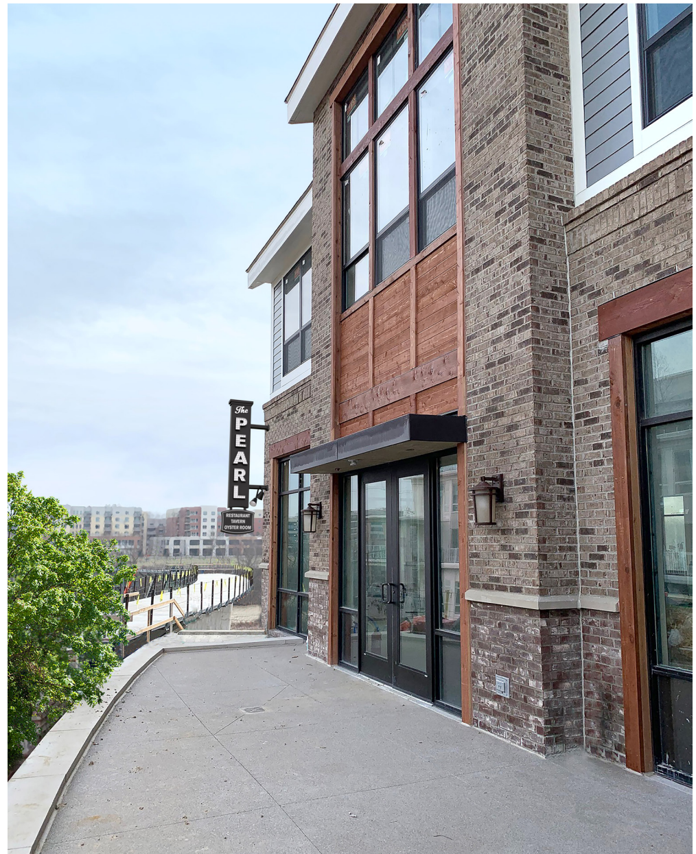
West Elevation | Day Time View
