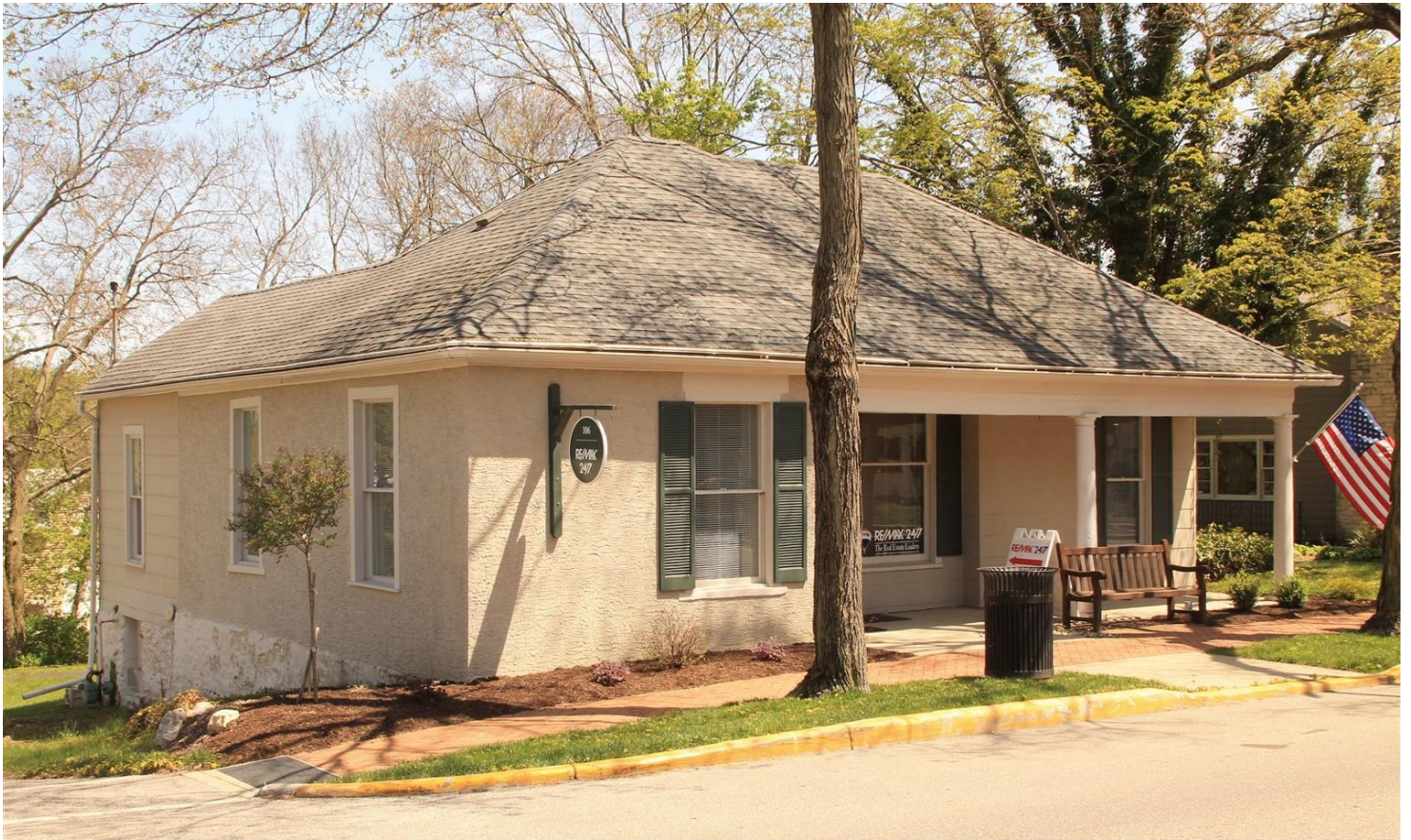
EXISTING BUILDING (WEST FAÇADE ON SOUTH HIGH STREET (ABOVE))
