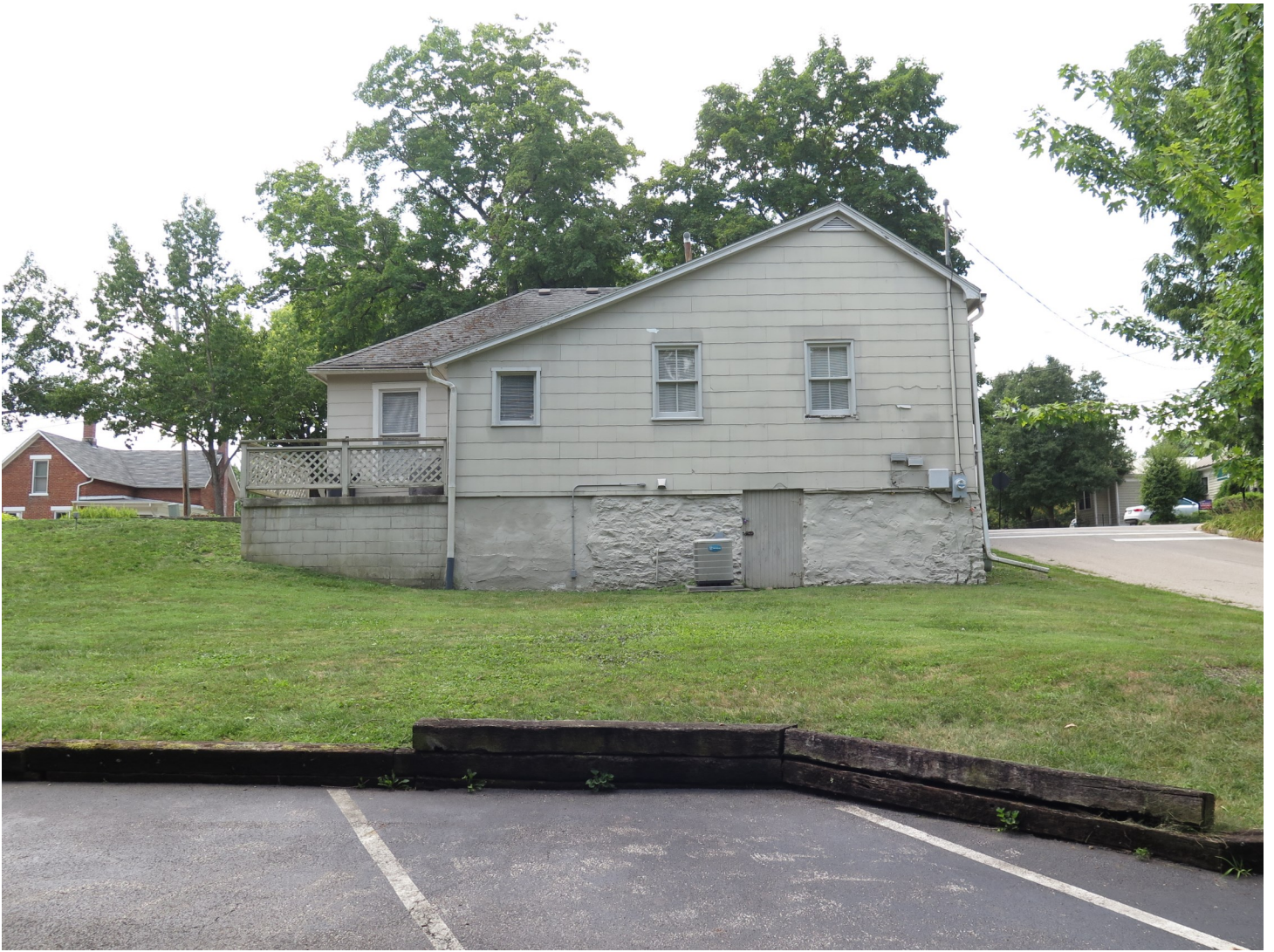
EXISTING REAR OF BUILDING FACING PARKING LOT (EAST FAÇADE)
