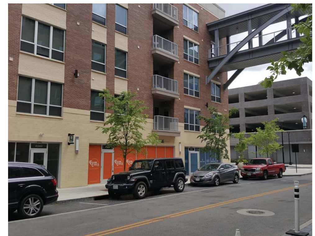
BRIDGE LOOKING SOUTH
