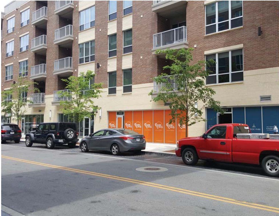
STOREFRONT LOOKING NORTH EAST
