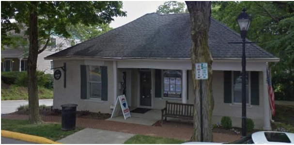
1. 106 S. High Street, west (front) side. (Source: Google Earth)
