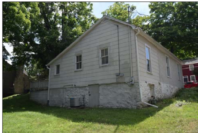
106 S High St, privy, looking southwest
