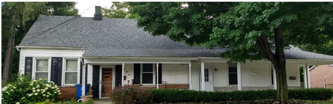
1. 156-158 S. High Street. The applicant proposes to demolish the non-contributing duplex and replace it with two single-family residences.
