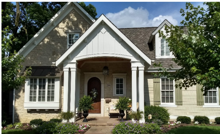
3. 200 S. High Street. The new single-family home was built in 2014 with traditional features such as the stone foundation, shingle siding, the stone-faced front gable with bay window, the front-gable porch with entry, and six-over-six sash windows with shutters and trim.
