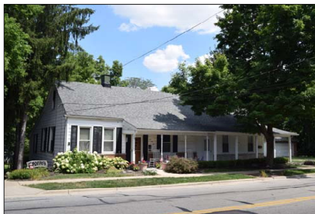
156-158 S High St, looking southeast
