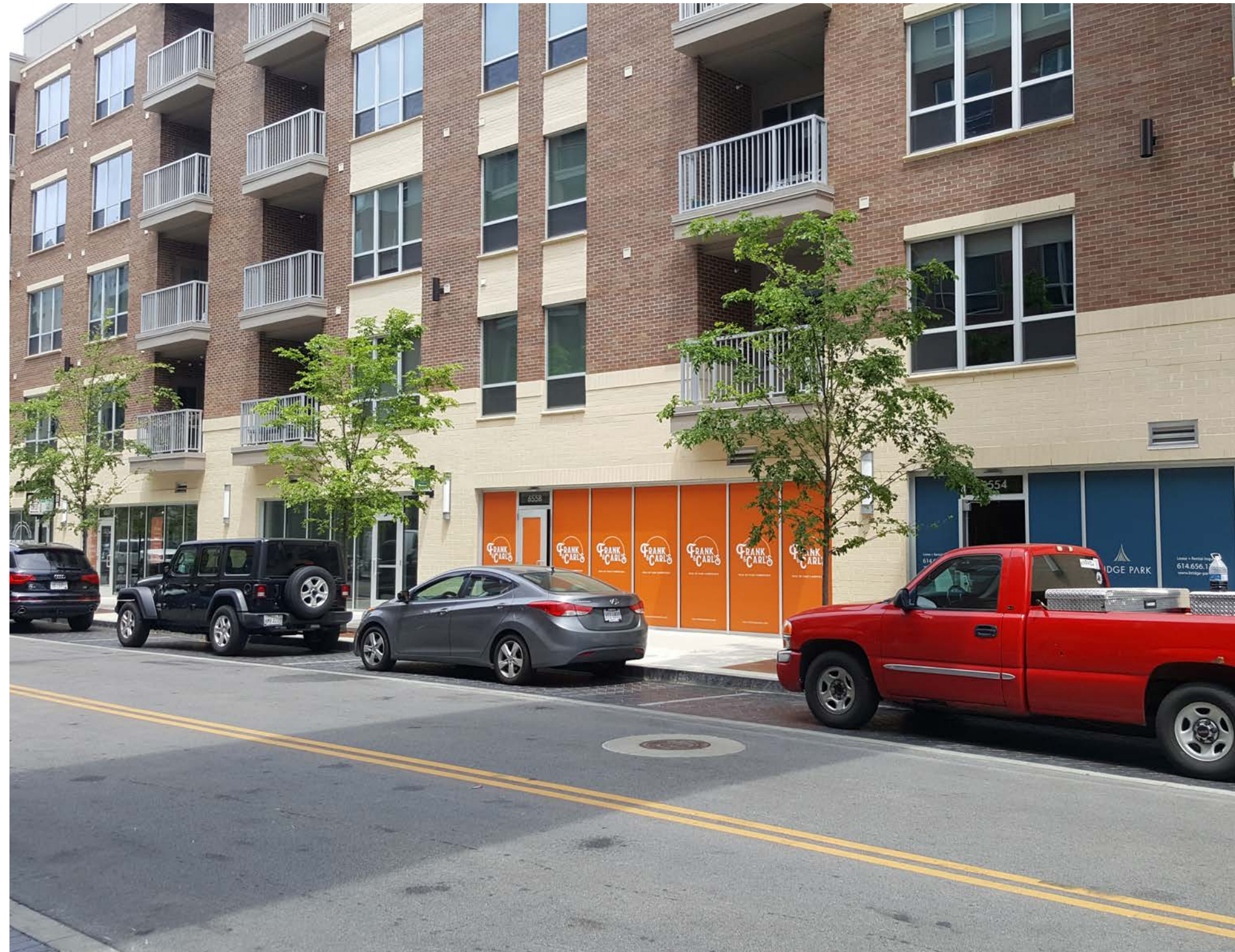
STOREFRONT LOOKING NORTH EAST
