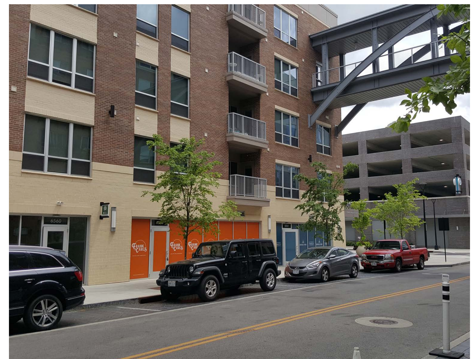
BRIDGE LOOKING SOUTH
