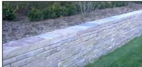
4 LIMESTONE ENTRY WALLS • MORTARED LIMESTONE WALL • RAKED JOINTS
