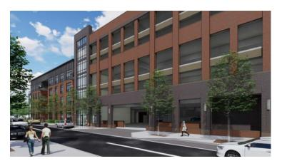
upper levels of the parking structure clad with red brick. At the wall openings, buff brick is applied horizontally as an accent along the floor line of the third and fifth levels, with a galvanized steel cable barrier system above.
