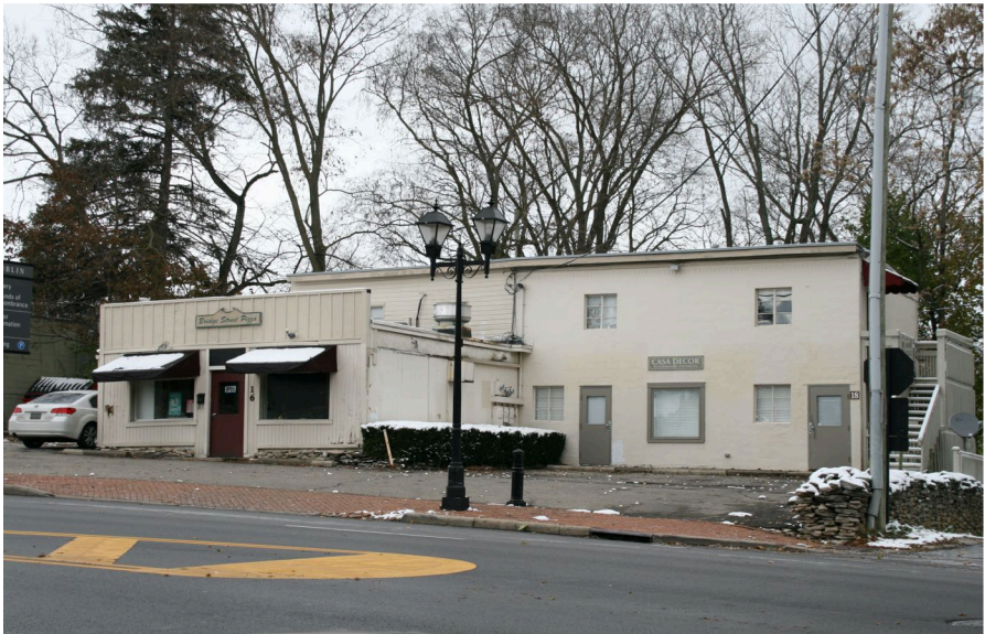
South East Facade
