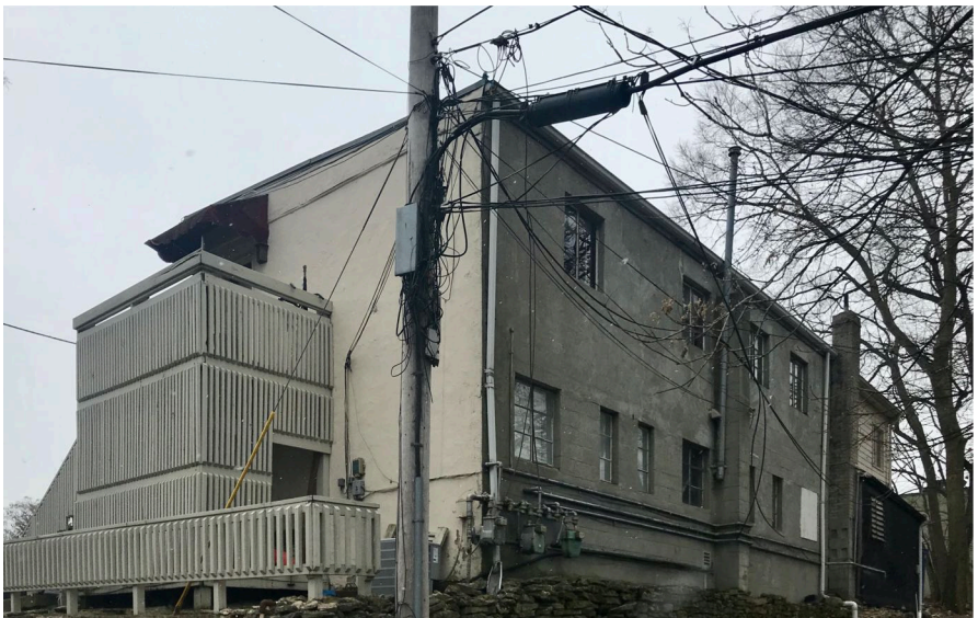
North East Facade
