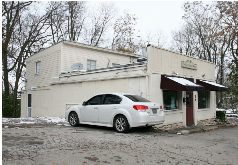
South West Facade
