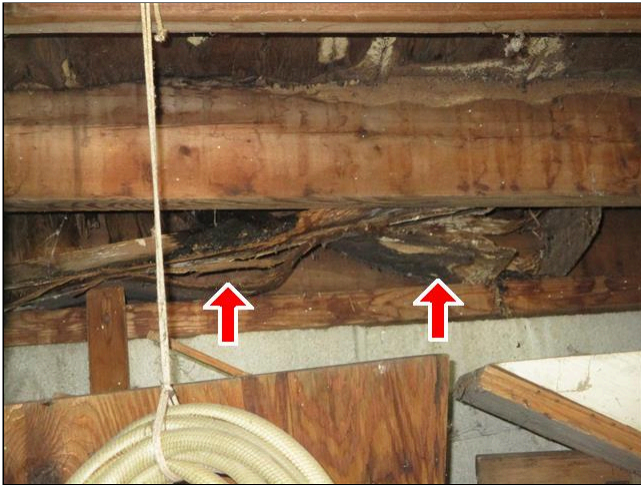
1.0 ROOF COVERING Picture 3
