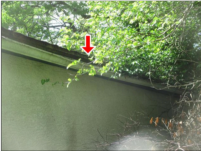
1.4 RAIN GUTTERS Picture 2
