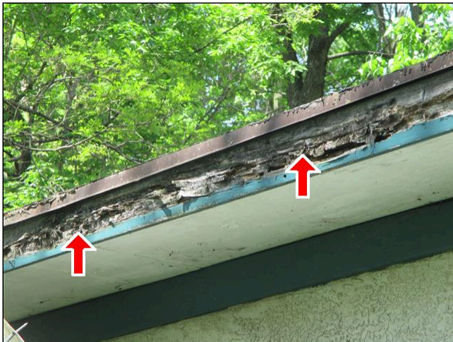
1.6 FASCIA / SOFFITS Picture 1
