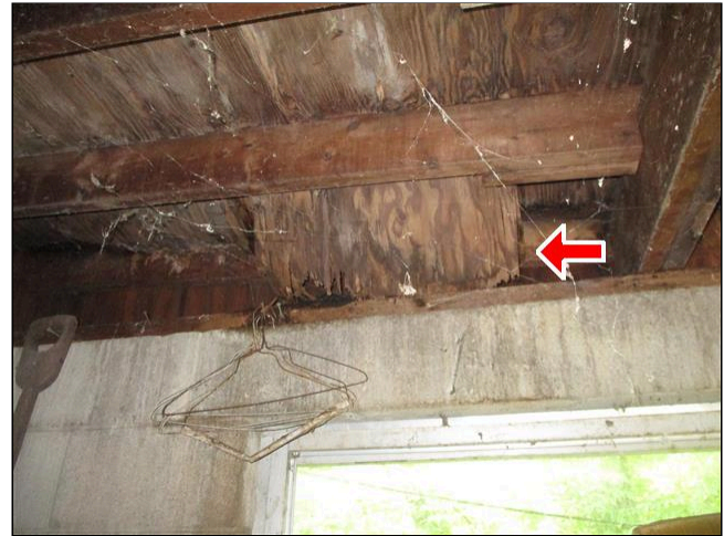
1.0 ROOF COVERING Picture 4
