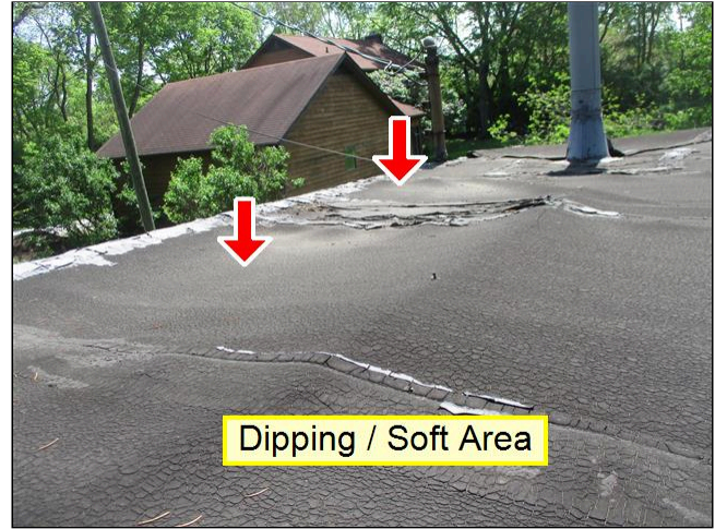
1.0 ROOF COVERING Picture 2
