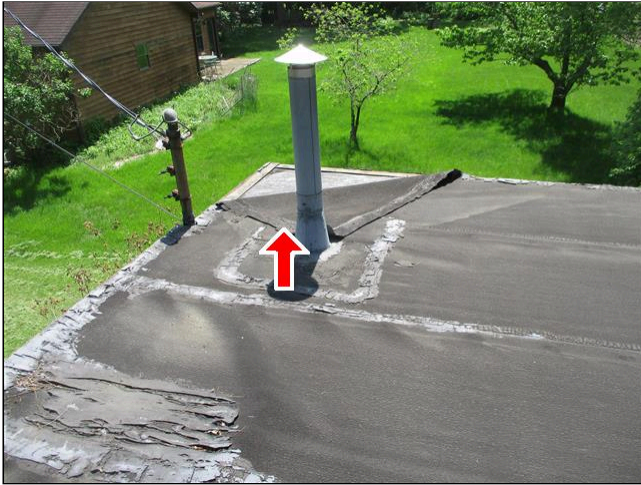
1.0 ROOF COVERING Picture 1
