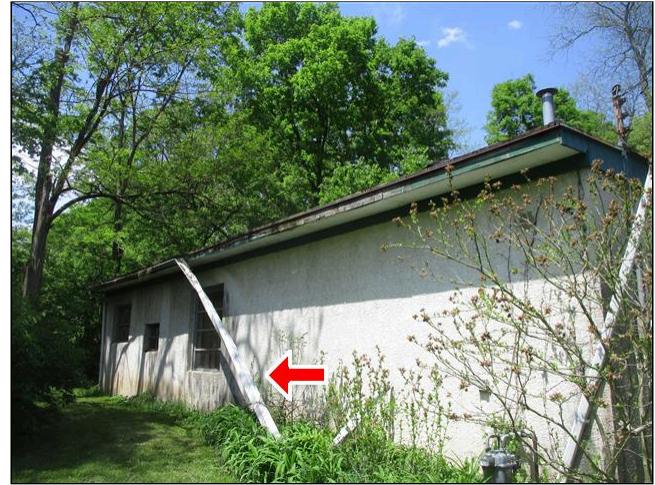
1.4 RAIN GUTTERS Picture 1
