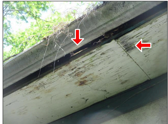
1.6 FASCIA / SOFFITS Picture 2
