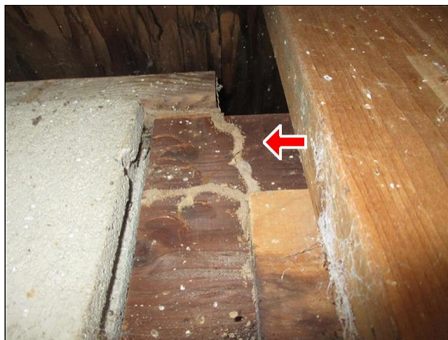
4.0 EXPOSED FRAMING Picture 1
