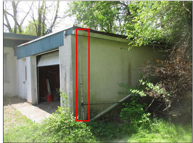
1.5 DOWNSPOUTS / ROOF DRAINS Picture 1
