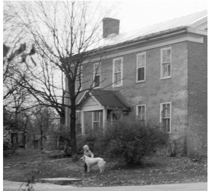
109 South Riverview Street, built ca. 1827, is an example of Federal architecture. Note the Federal-style elements such as the two-story height, rectilinear form, five-bay façade composition with symmetrical window and door placement, and a side-gable roof.
