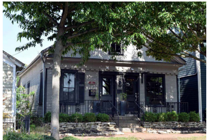
87 South High Street, built ca. 1840, in a Greek Revival architectural style has a rectilinear footprint with stone foundation, front gable façade clad in horizontal siding accented by a decorative frieze.
