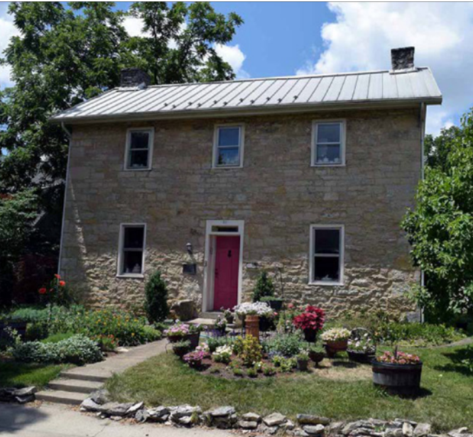
83 South Riverview Street, built in 1824, is an example of an I-House building type with Federal architectural style elements. The building is of stone construction with a standing seam metal roof.
