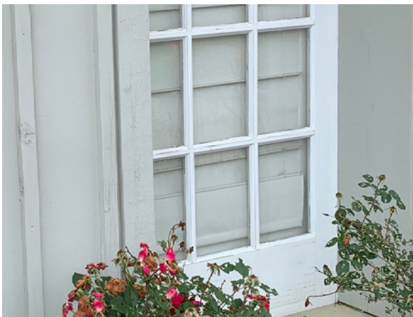
Real divided lite window, 31-33 South High Street
