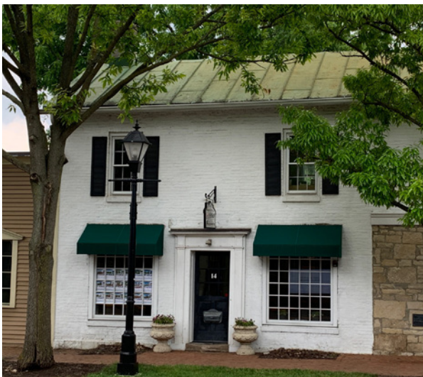
Commercial storefront, 14 South High Street
