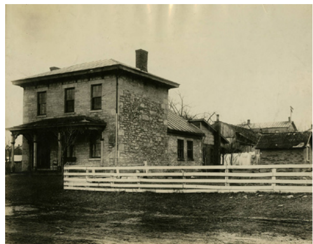
Home of Isaac Walter, 37 South Riverview Street, 1842
