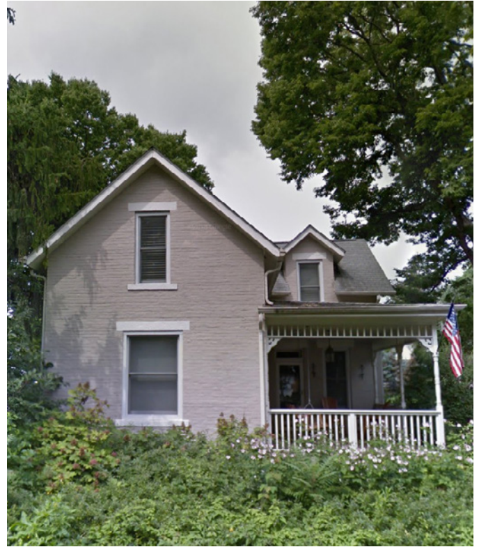
55 South Riverview Street, built ca. 1900, is an example of the Gabled Ell building type with No Academic Style. The front block and wing are identifying forms with the spindle work suggesting an increased accessibility of millwork at the turn of the century.
