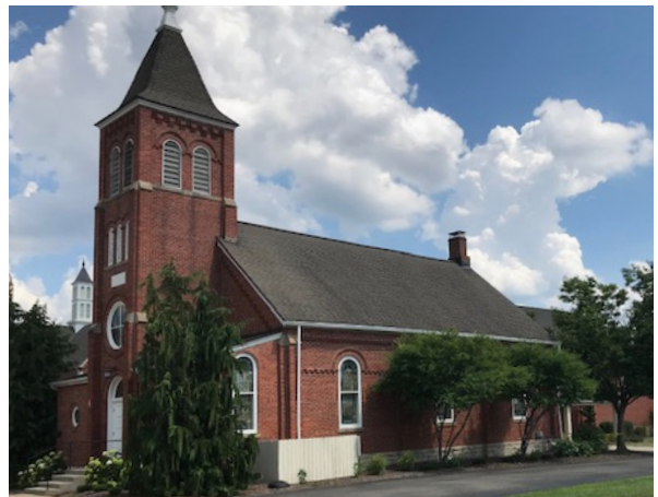
St. John Lutheran Church, 6115/6135 Rings Road
