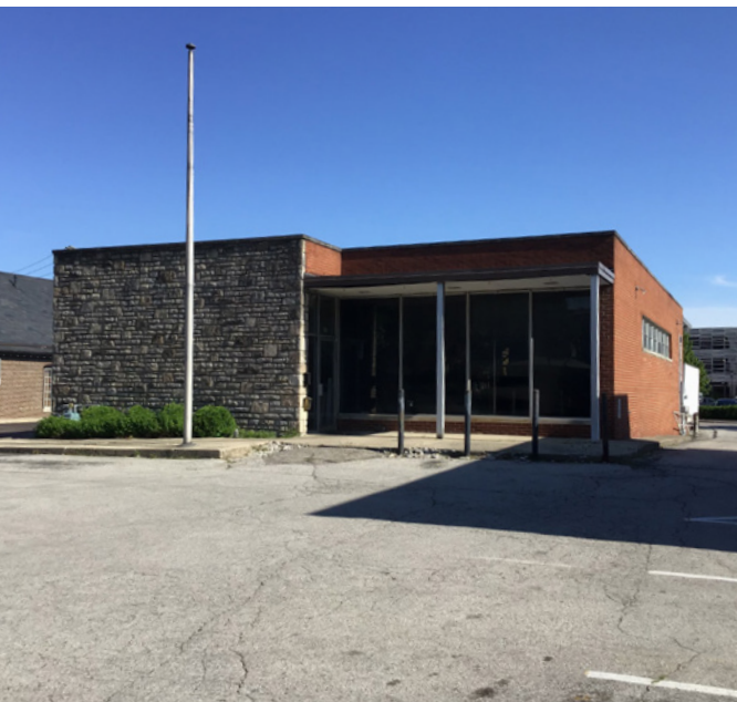
The former Post Office at 38 West Bridge Street, built in 1965 is in a Modernist Movement architectural style. The one-story brick and stone building has a rectilinear footprint with flat roof and a large glazed storefront window.
