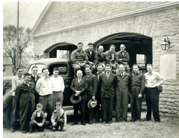
Dublin Firehouse, 37 West Bridge Street, 1945
