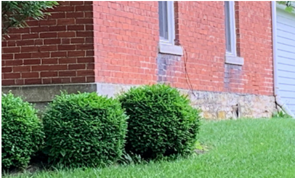
Original stone foundation, 167 South High Street
