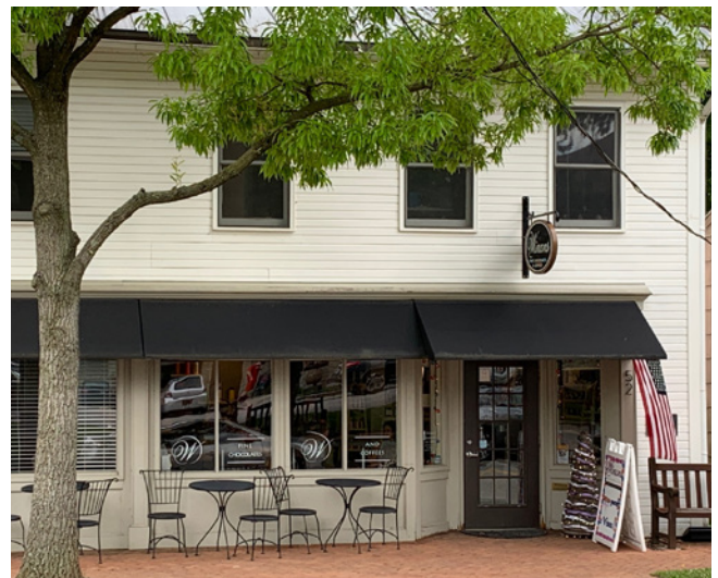
Recessed entry and bulkheads, 52 South High Street
