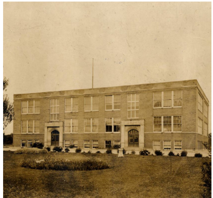
The Washington Township Centralized School at 150 West Bridge Street, built in 1919 in the Art Deco style. Elements of the style include the smooth wall surface and decorative concrete panels with stylized or geometric motifs.
