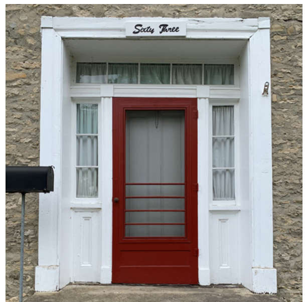
Original storm door, 63 South High Street
