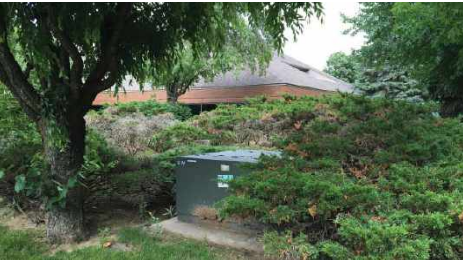
Existing landscape is often overgrown creating a "tired" appearance.
