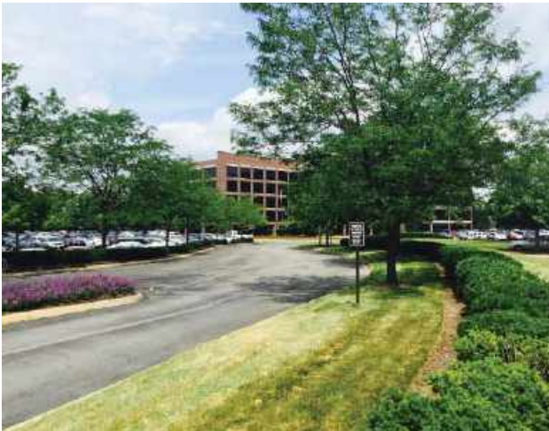
Individual entryways for different buildings, while often attractive, typically create great inefficiencies in the parking layout without mitigating issues within each site.
