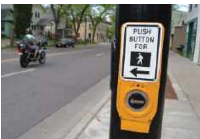
Automated pedestrian crossing signal
