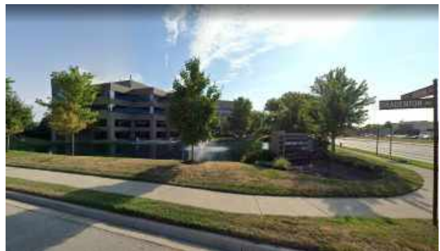
Existing 5080 Tuttle Crossing Blvd
