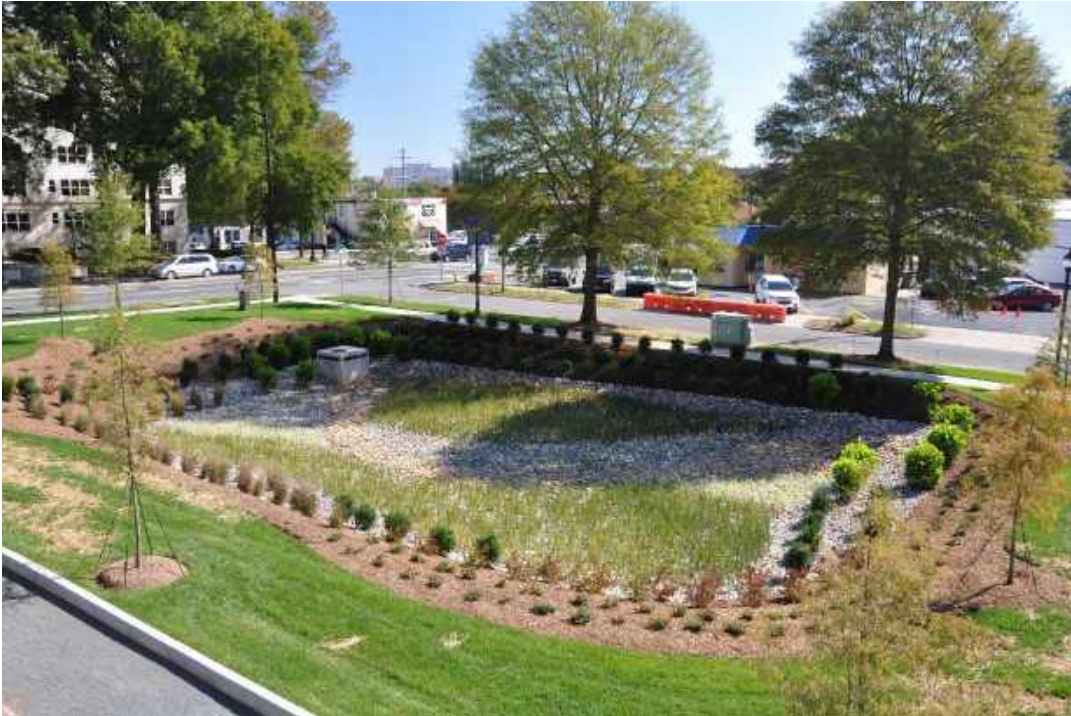
Example of a stormwater wetland integrated into a site design
