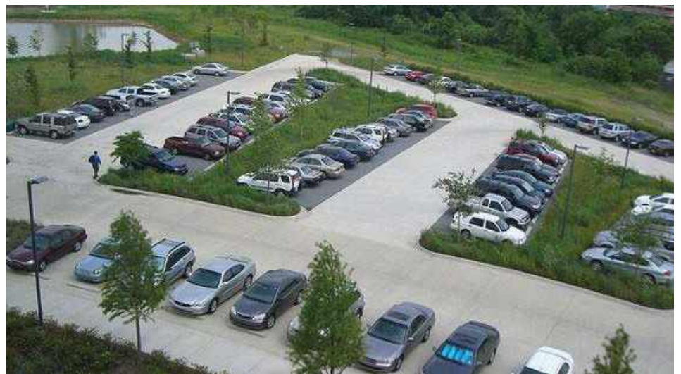
Parking lot stormwater approach: Curb breaks to accommodate inlet flow; large central islands
