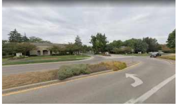
Existing Millennium Offices
