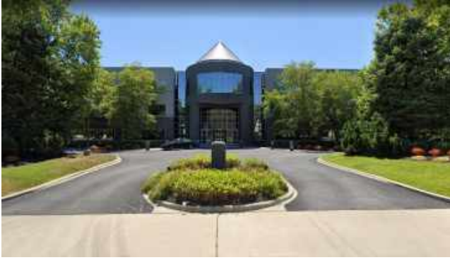
Existing Metro Center Office Building
