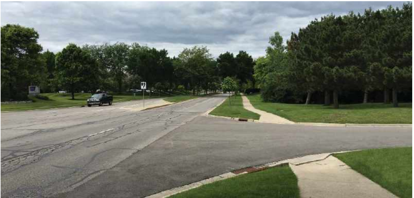
Existing medians limit opportunities for pedestrian crossings
