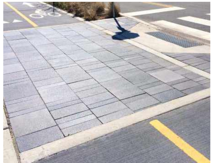
Examples of crosswalks with ornamental paving
