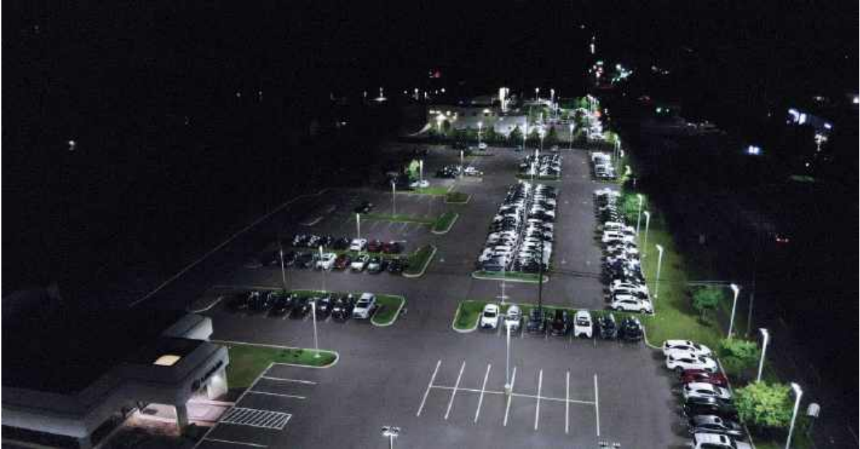
Example of Lighting in Parking Lot
