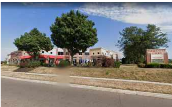
Existing Parkcenter Circle (development in City of Columbus)
