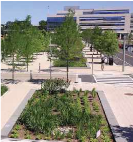
Tuttle/Rings: Central open space walkway
