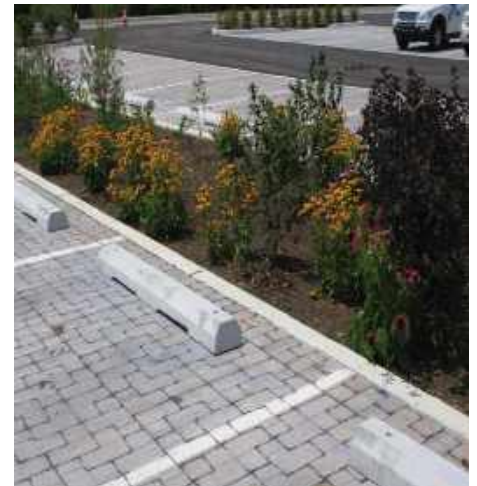
Permeable pavers in parking area
