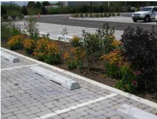
Permeable Pavers in Parking Area
