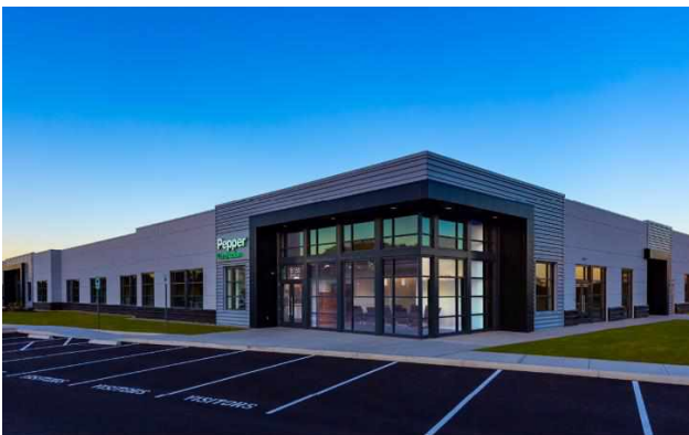
Examples of Building Designs that include a variety of elements including multiple materials, transparency, recesses and projections, and articulated entrances
