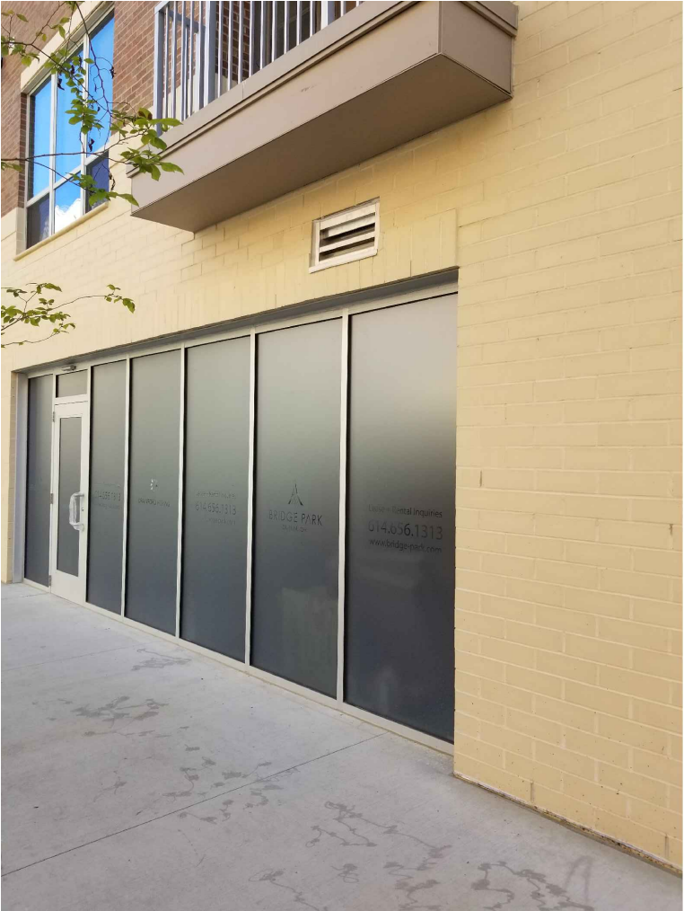
NORTH EAST VIEW OF EXISTING STOREFRONT
