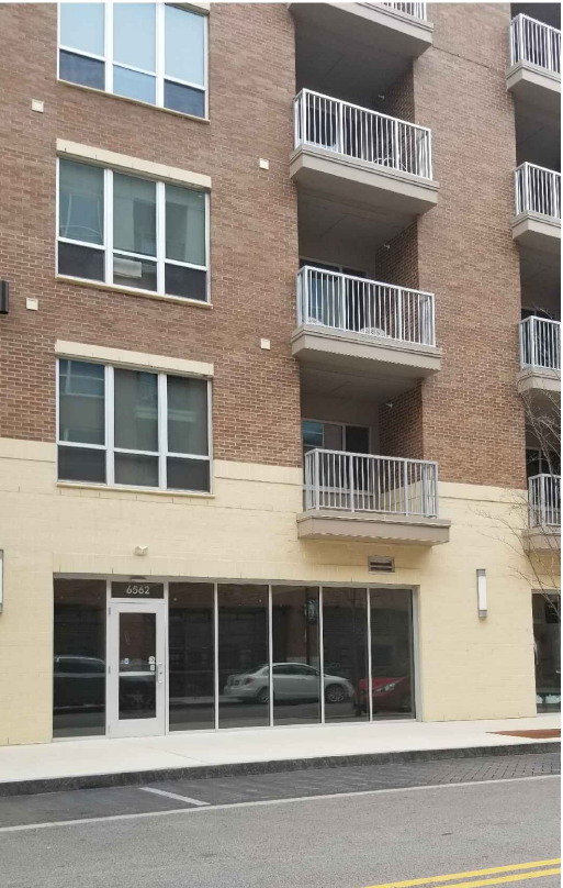
SOUTH EAST VIEW OF EXISTING STOREFRONT
