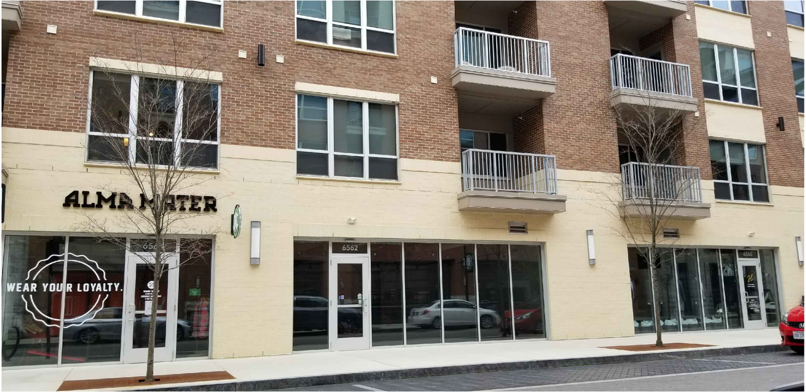
SOUTH EAST VIEW OF EXISTING STOREFRONT
