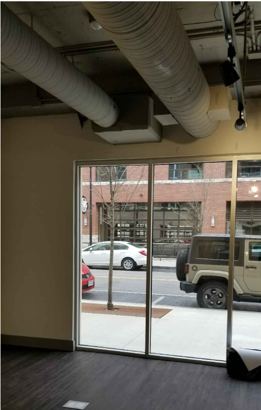
SOUTH WEST INTERIOR VIEW OF EXISTING STOREFRONT
