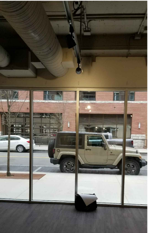
SOUTH WEST INTERIOR VIEW OF EXISTING STOREFRONT
