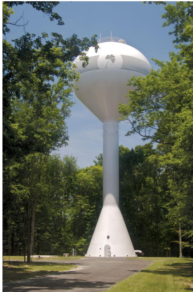
Tartan West Water Storage Tank (.5 MG)
