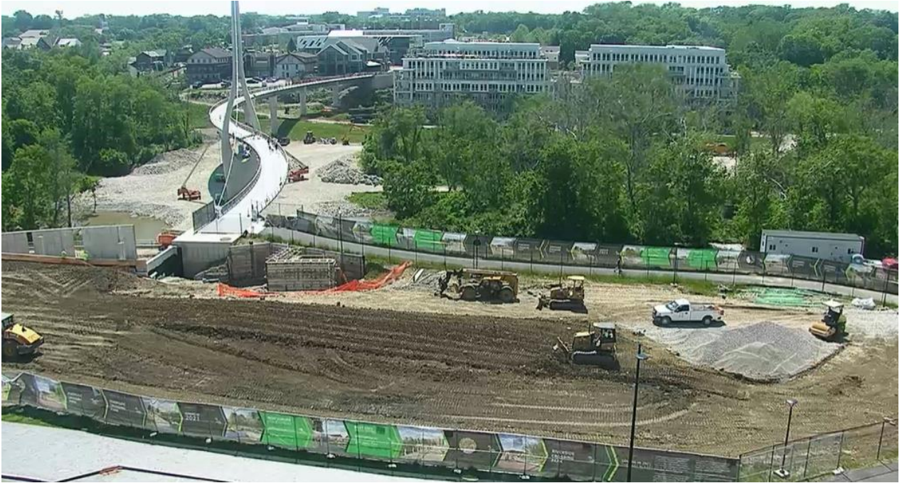
Riverside Crossing Park East Plaza construction as of June 2, 2020
