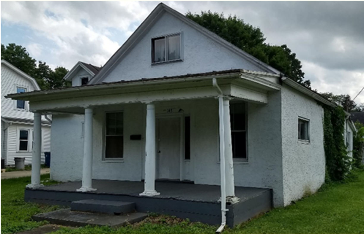
1. 143 S. High Street. The building to be demolished and replaced with the proposed dates to ca. 1890 and is recommended contributing to the City of Dublin's Historic District as well as the Dublin High Street Historic District National Register boundary increase. Traditional elements include the stone foundation, the full-length shed-roof front porch with a seam metal roof and Tuscan columns, and the large gable front covered with a seam metal roof.
