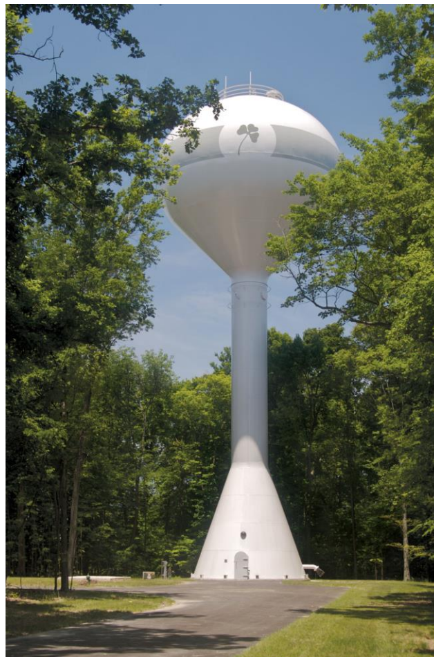
Tartan West Water Storage Tank (.5 MG)
