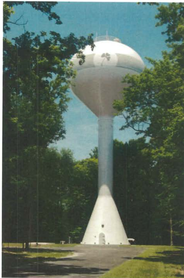
Tartan West Water Storage Tank (.5 MG)
