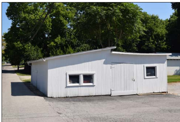
119 S High St, storage building, looking northeast
