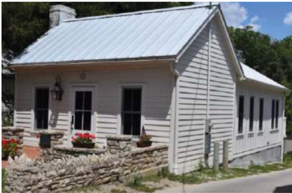
2. 38 S. High Street. The one-story wood-frame structure dates to ca. 1850 and is listed on the National Register as part of the Washington Township MRA. It is also recommended contributing to the City of Dublin's Historic District and the Dublin High Street Historic District National Register boundary increase. The building resembles a hall-and-parlor structure with its horizontal clapboard siding. (Individual Property Sheet, City of Dublin Historical and Cultural Assessment).
