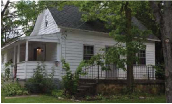
1. 37 N. Riverview Street. The wood-frame dwelling dates to ca. 1850. The house has a hall-and-parlor plan and is clad in clapboard siding, including the shed-roof addition to the left of the main house. (Individual Property Sheet, City of Dublin Historical and Cultural Assessment).
