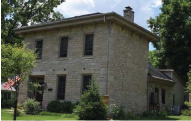
4. 37 S. Riverview Street. This Italianate-style house dates to ca. 1855 and is of coursed ashlar stone masonry construction. Note the stone head and sills of the windows on the façade. Details such as these should be used as inspiration for new construction in the historic district. (Individual Property Sheet, City of Dublin Historical and Cultural Assessment).
