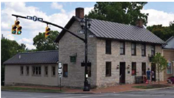
3. 6-12 S. High Street. This Federal-style building dates to 1832 and is of coursed ashlar stone masonry construction. Window details such as these should be used as inspiration for new construction in the historic district. Also note the one-story addition to the rear of the structure clad in horizontal siding. (Individual Property Sheet, City of Dublin Historical and Cultural Assessment).
