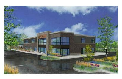
cementitious horizontal siding (Cobblestone), and two finishes of metal panels (SW 7740 Messenger Bag and Aged Copper) as secondary materials.
