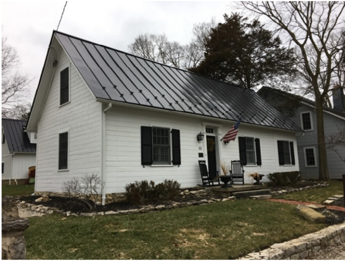
Figure 6. 63 S Riverview St. This house is an example of a one-and-a-half house. Note the horizontal siding and sash windows. (Preservation Designs, March 2021)
