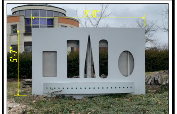
EXISTING SIGN TO BE REMOVED
