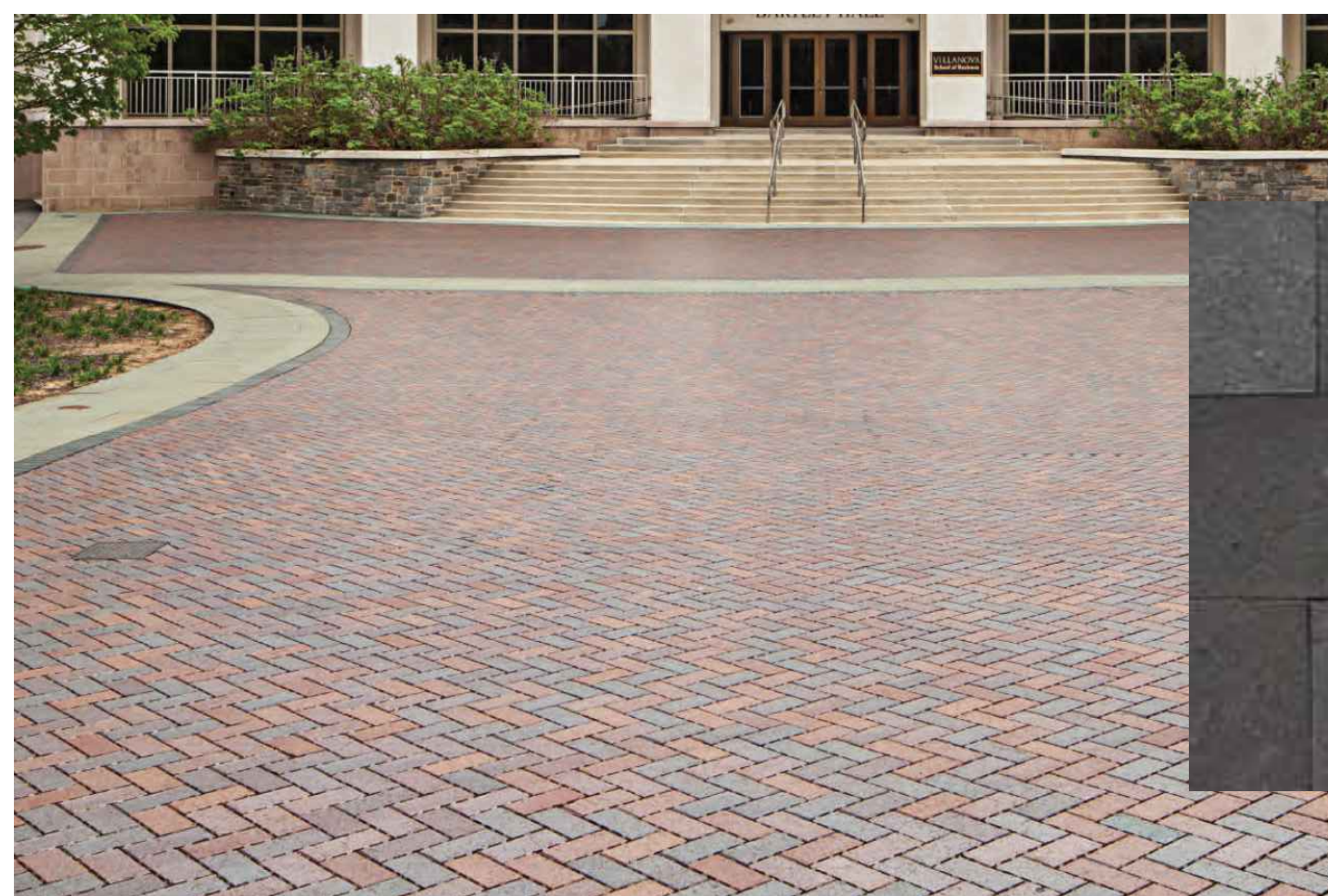
AVAILABLE FROM ENDICOTT CLAY PRODUCTS CO., 2 1/4" x 4" x 8", LAID IN A HERRINGBONE PATTERN, MANGANESE IRONSPOT IN COLOR.
