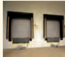
Rolling Service Doors
