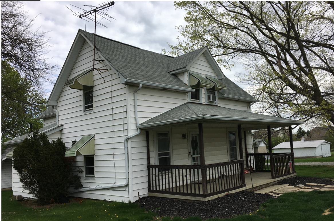
1. Farmhouse at 7298 Post Road, looking northeast.
