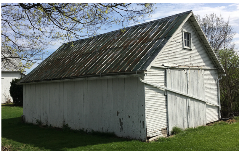
12. Looking north by northeast at the granary.
