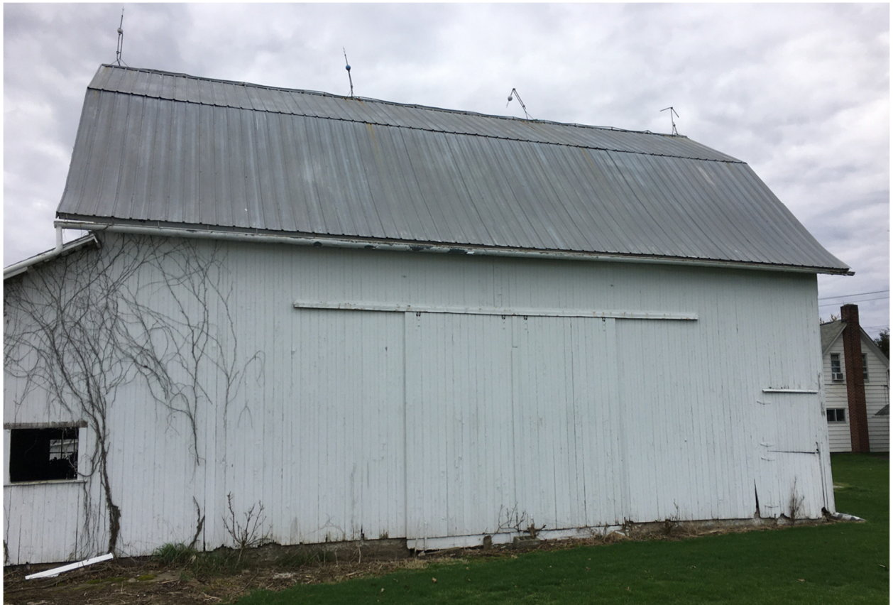
7. View of barn's north elevation.
