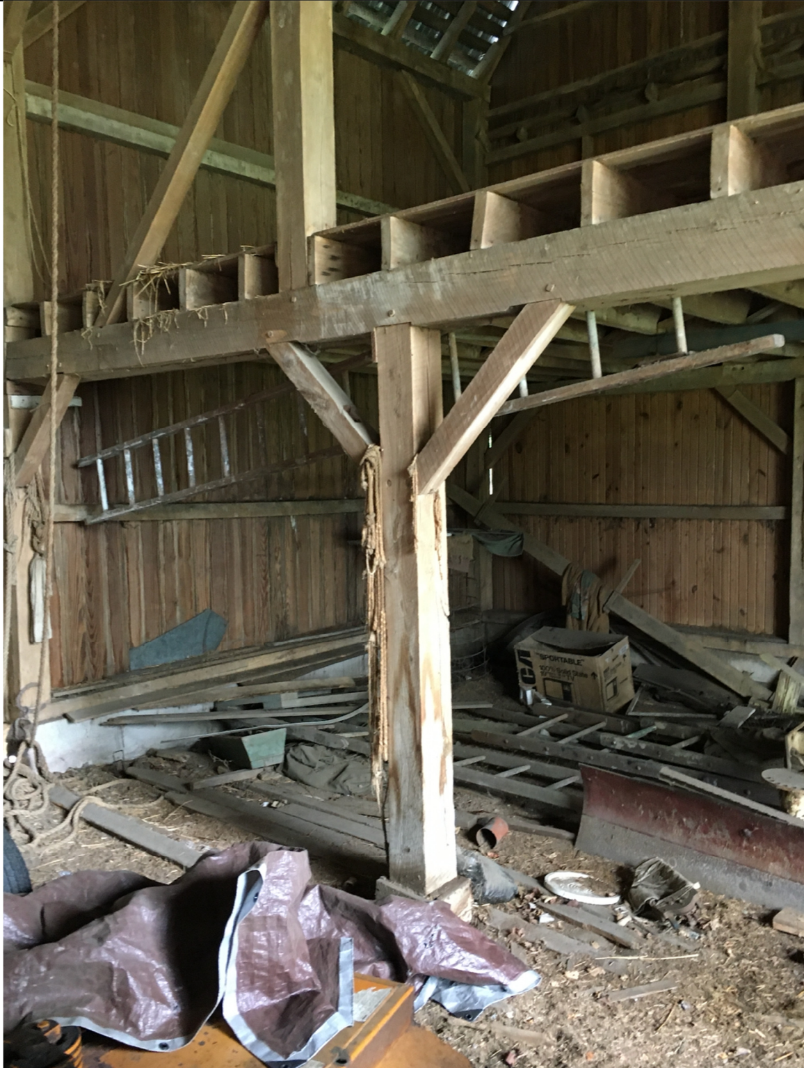
9. Interior view of barn, showing traditional wood joinery of mortise and tenon secured with wooden pegs. Note the circular marks on the heavy timbers from the saw mill.
