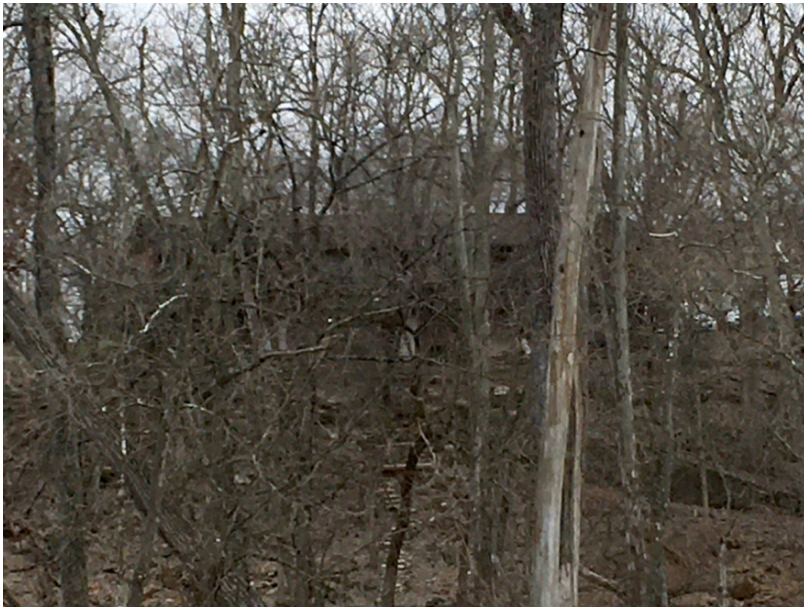
Figure 5. 110-112 S. Riverview Street taken from across the Scioto River. While much is obscured, this photo shows the existing access paths down to the river. The proposal should address site issues such as existing landscape features which will be maintained or removed (Preservation Designs, March 2021)
