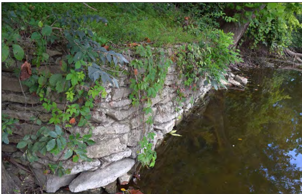
Figure 89. Dry-laid stone wall in general vicinity of the Joseph Corbin Stone Mill, looking northwest
