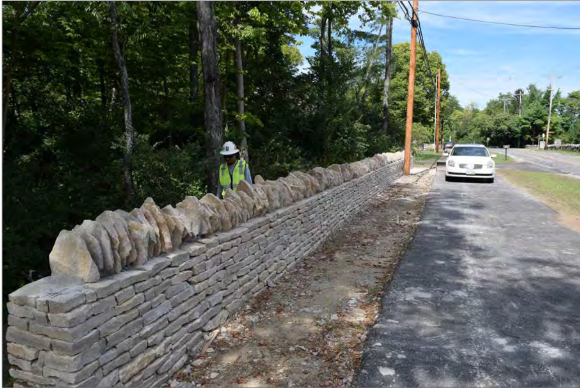
Figure 96. Wall in process of being rebuilt as part of trail project (W034 along west side of Dublin Road south of downtown, looking north). Note top course set in mortar.
