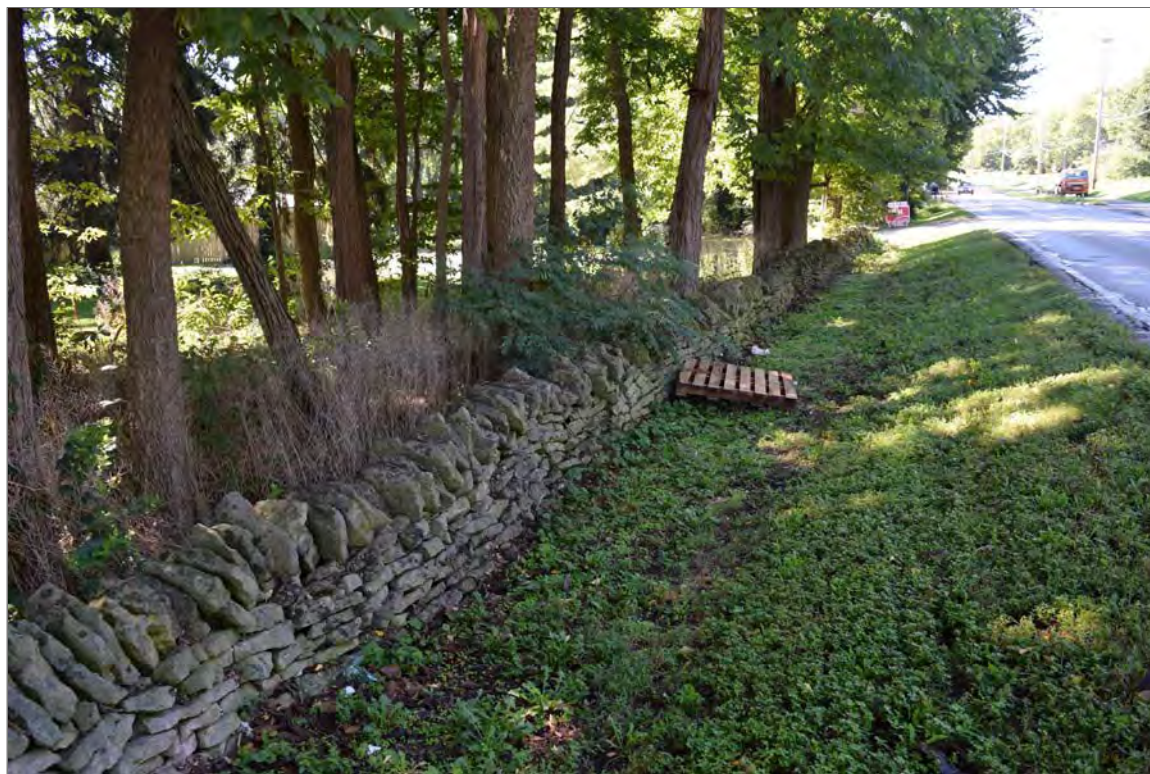
Figure 92. Example of lower wall with slightly smaller stones (Wall W033 along Riverside Drive, looking south)
