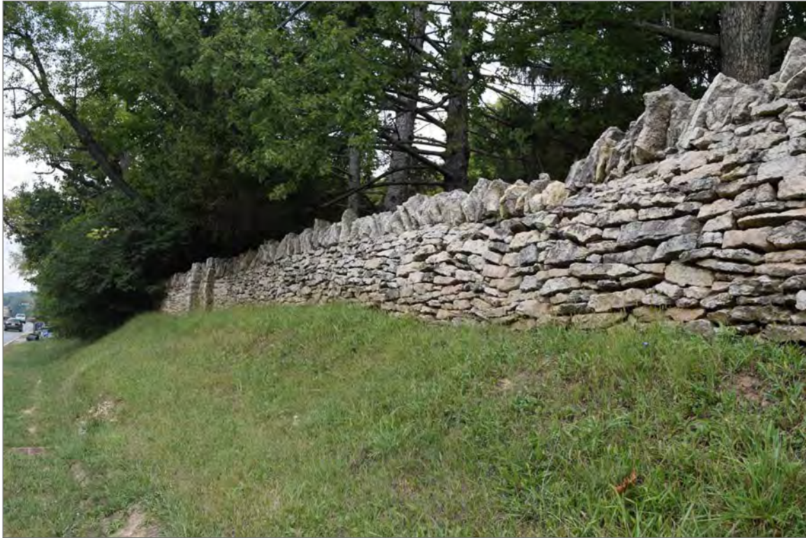
Figure 93. Example of taller wall with larger stones (Wall W005 along Riverside Drive, looking north)
