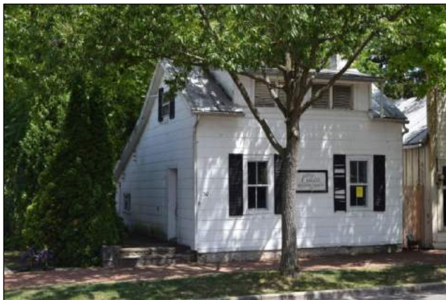
30 S High St, looking southeast
