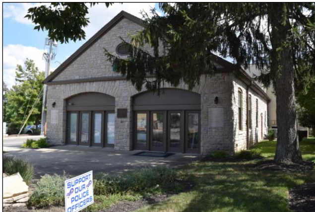
37 W Bridge St, looking southeast
