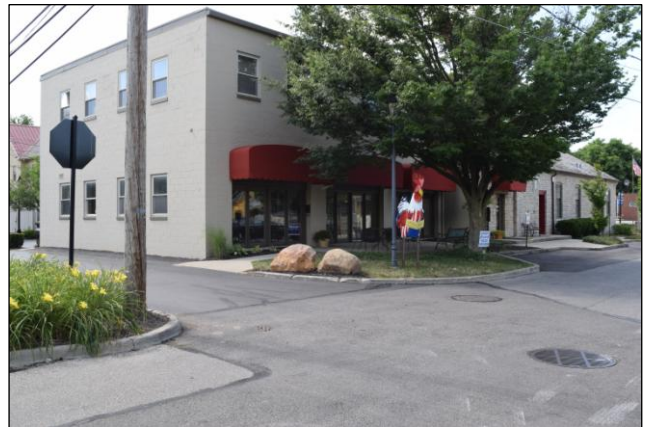
37 W Bridge St, looking northwest
