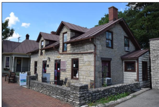
16 N High St, looking northeast
