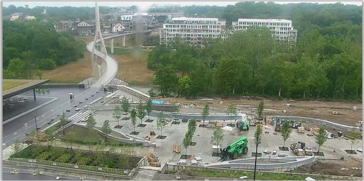
Riverside Crossing Park East Plaza construction as of July 2021
