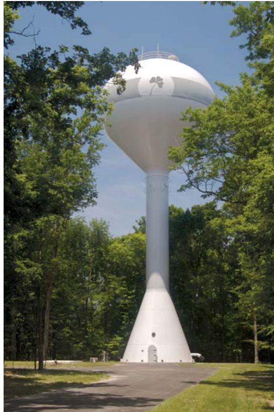
Tartan West Water Storage Tank (.5 MG)
