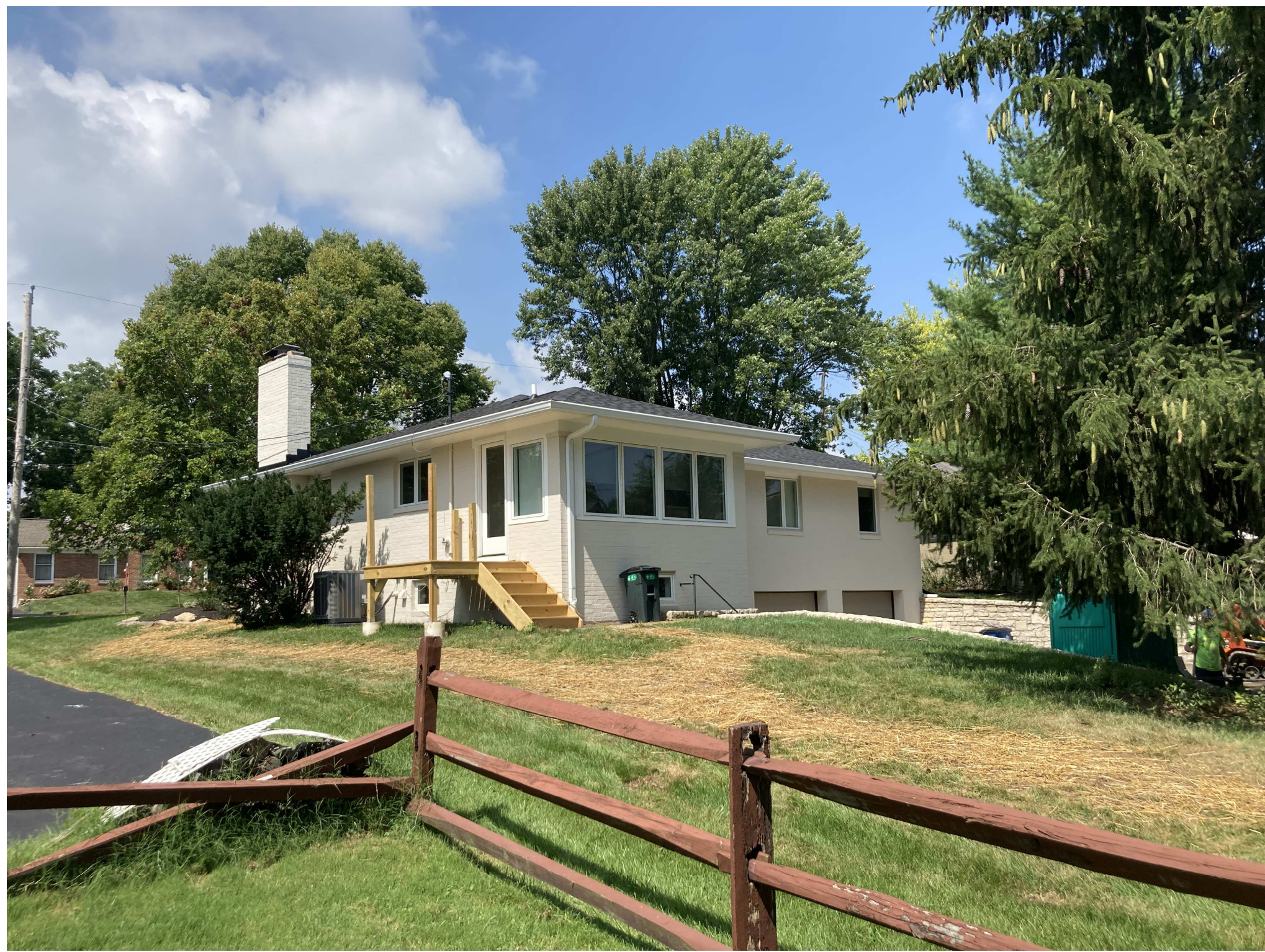
86 FRANKLIN STREET - REAR VIEW NORTHERN ADJACENT PROPERTY
