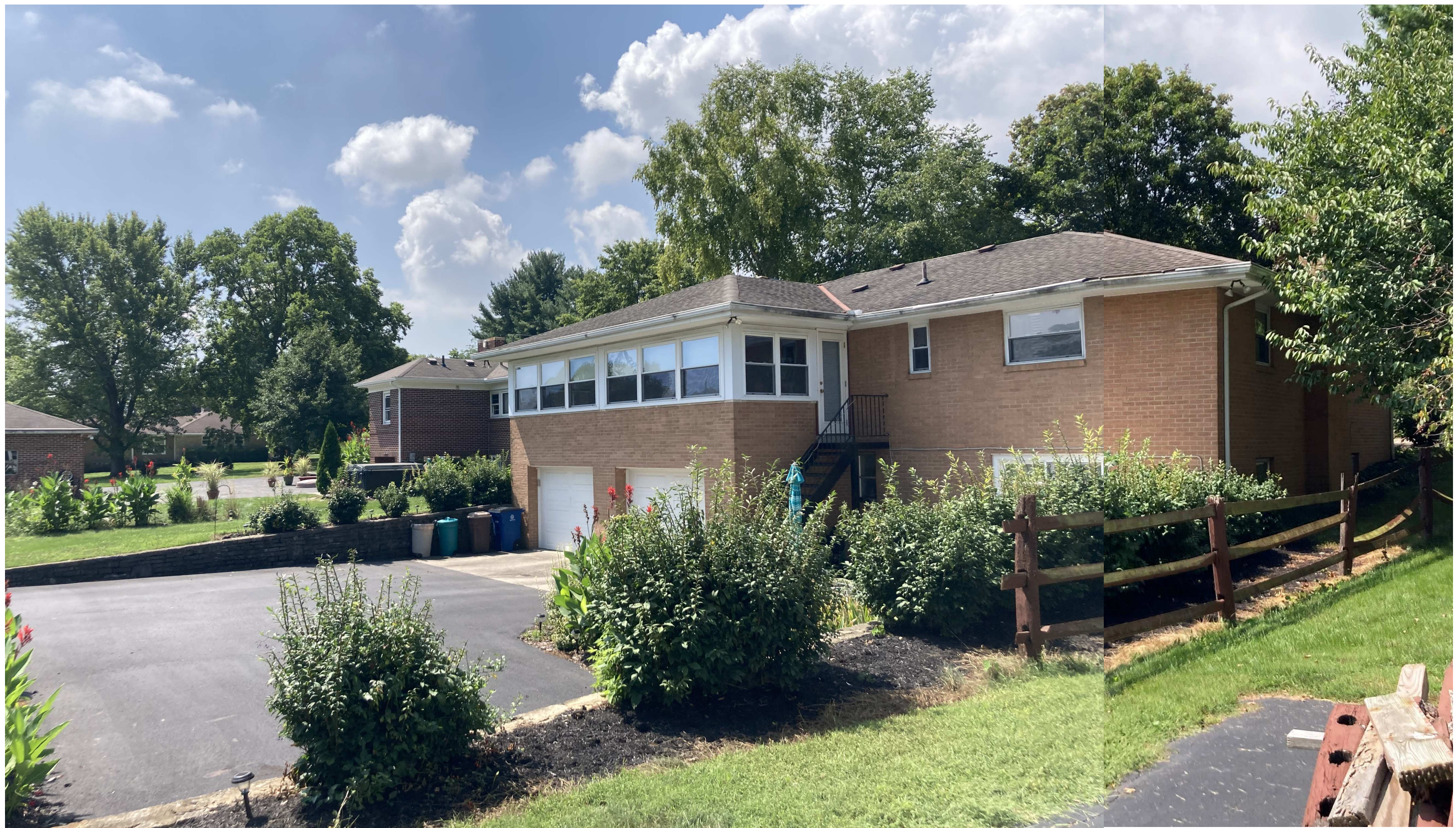
100 FRANKLIN STREET - REAR VIEW SOUTHERN ADJACENT PROPERTY
