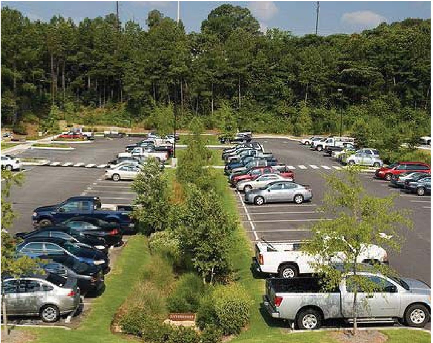
Parking lot stormwater approach: Bioswale and large central island
