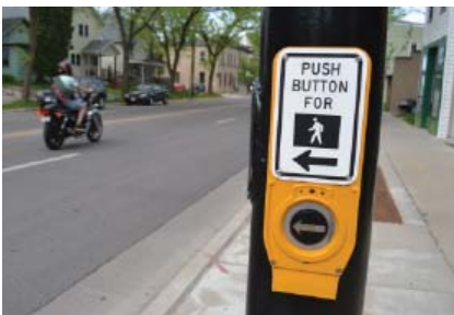
Automated pedestrian crossing signal
