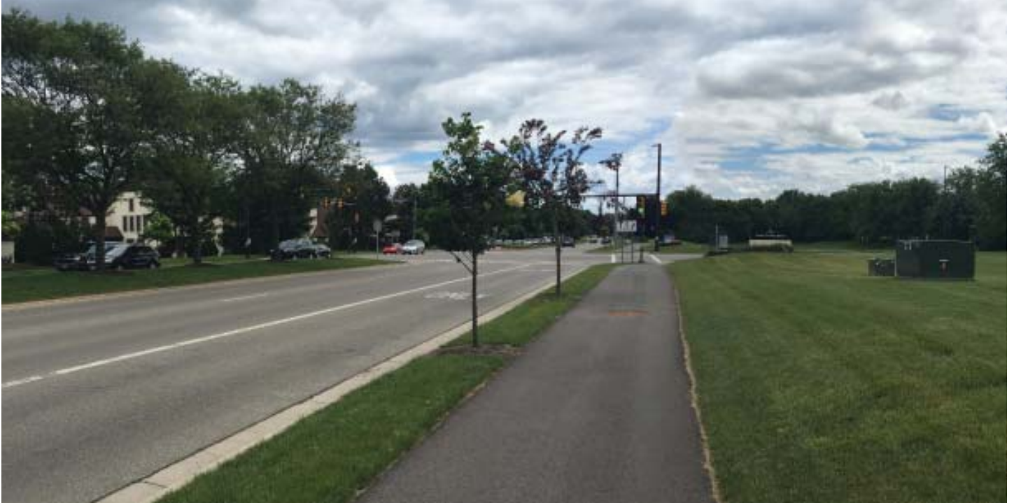
Frantz Road and Metro Place South - EXISTING
