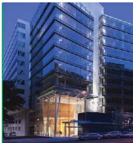
Extensive use of glass as exterior material
