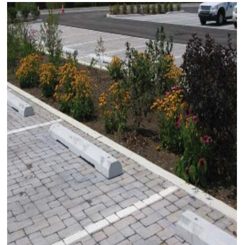
Permeable pavers in parking area
