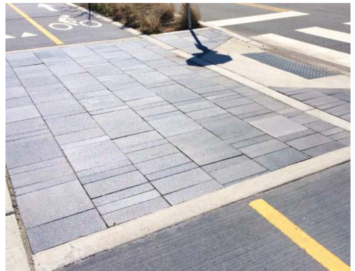
Examples of crosswalks with ornamental paving
