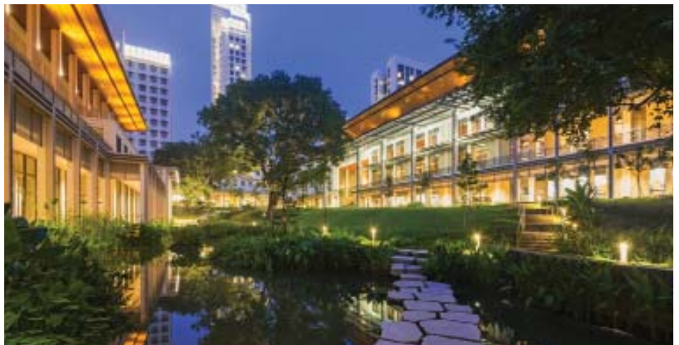
Glass and metal as exterior building materials; high degree of transparency
