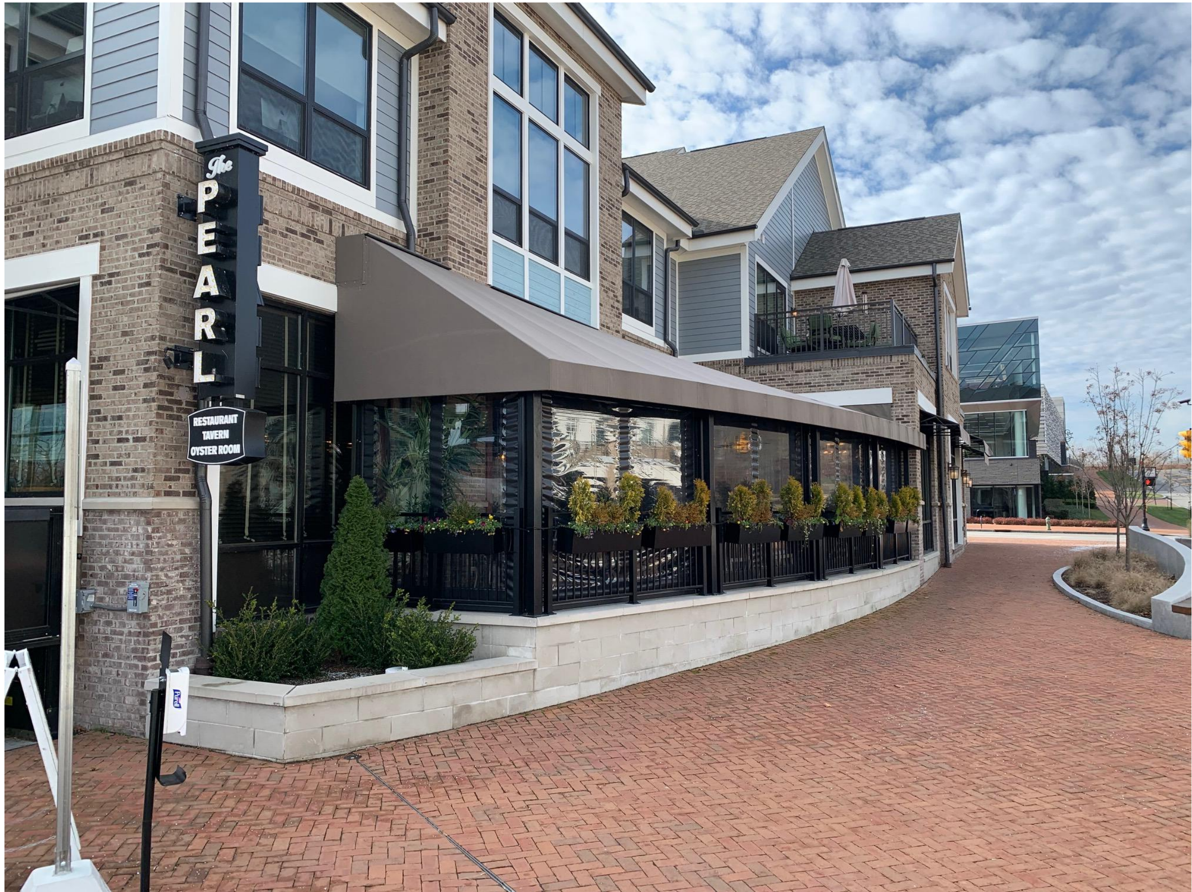
VIEW LOOKING SOUTHWEST
