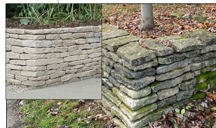
Dublin - Shoreline stone wall 3-5" thk, cut & faced to 8-16" w x 9-24" length (buff-grey, natural product, procured from site and Lang Stone Co.)
