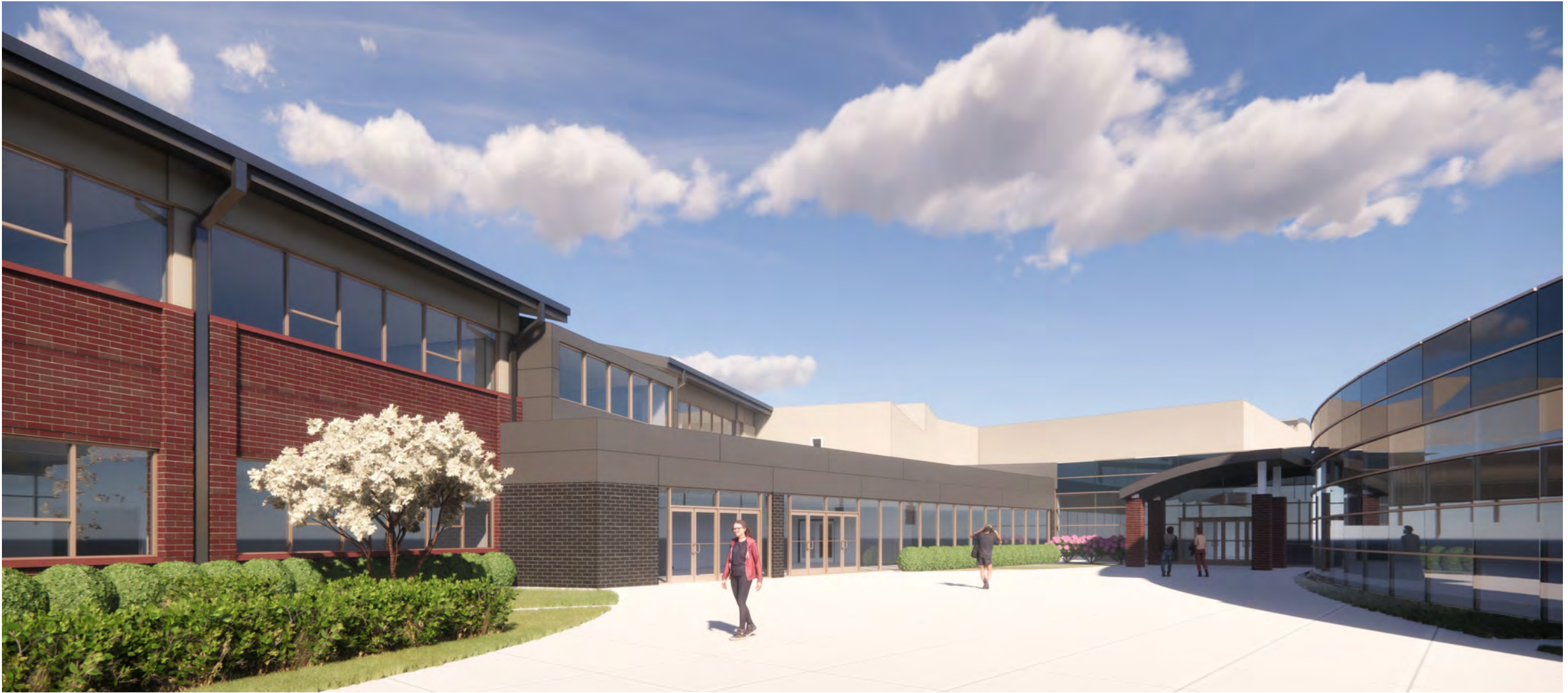
View of south entry
