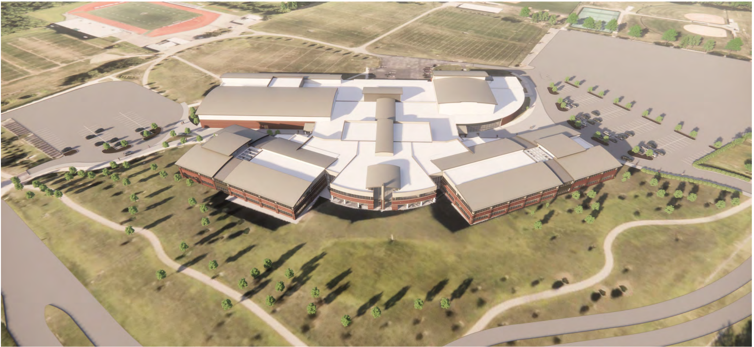
Aerial view from intersection
