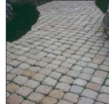
Lannon tumbled cobbles (buff grey, natural limestone product, procured from Lang Stone Co.)
